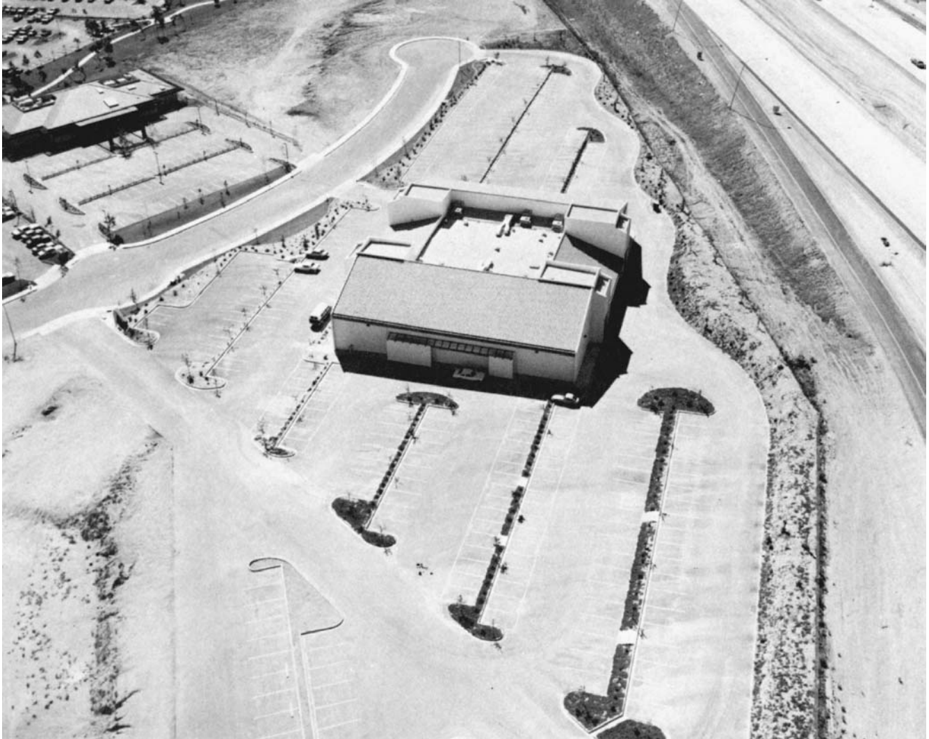
Figure 19.61 Aerial photo of finished roof. (William Boggs Aerial Photography. Reprinted with permission.)
