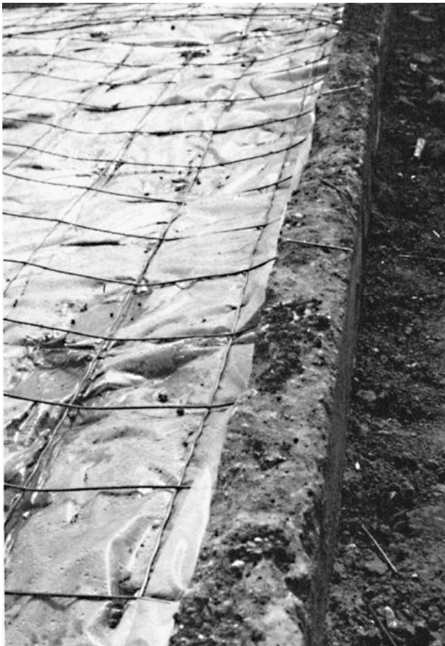
Figure 9.11 Reinforcing mesh and plastic.
