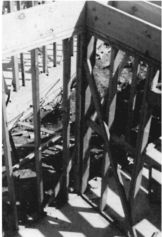
Figure 10.15 Intersection of exterior wall and interior wall.
