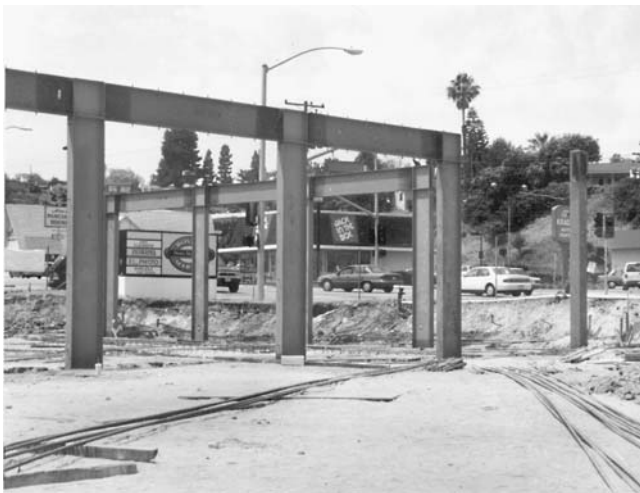
Figure 7.27 Photograph ground floor steel columns and beam.
