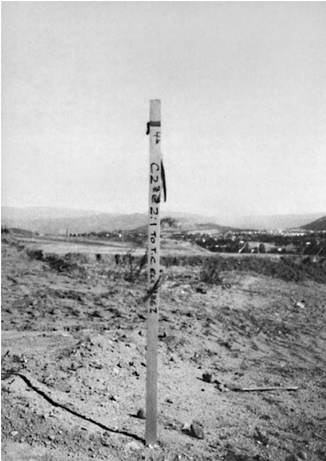
Figure 19.14 Stakes placed by surveyor.
