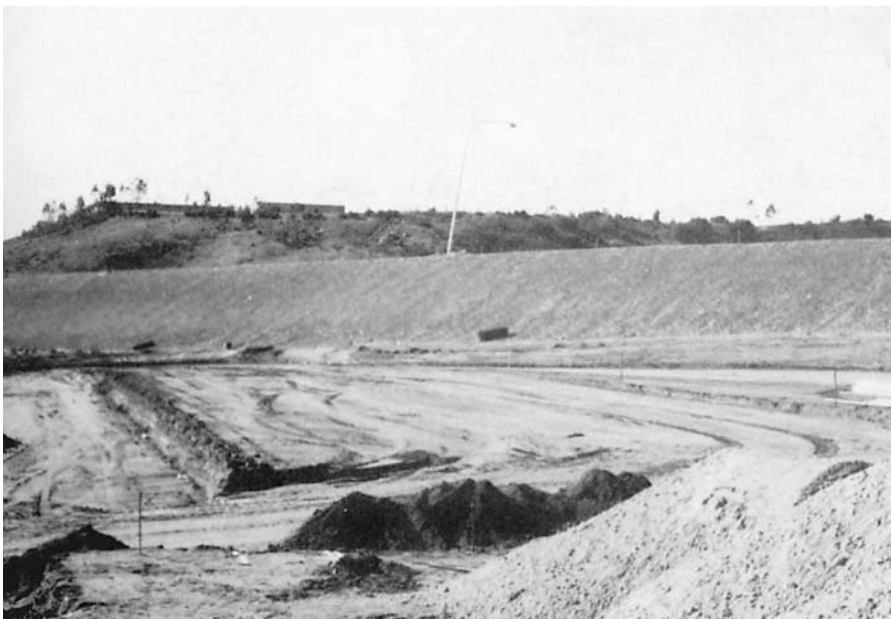
Figure 19.13 Grading the property.
