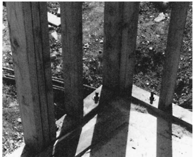
Figure 10.12 Corner at sill.
