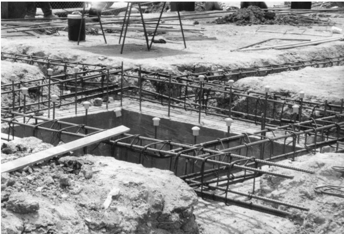
Figure 20.46 Formwork for concrete spread footing at steel columns.
