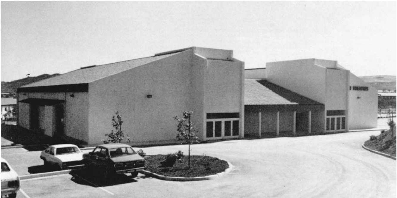
Figure 19.46 Rear view of finished structure.
