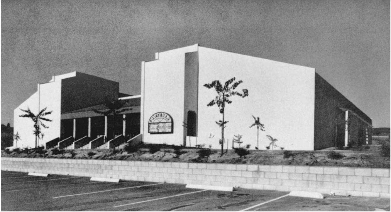
Figure 19.45 Front view of finished structure. (Photography: Kent Oppenheimer.)
