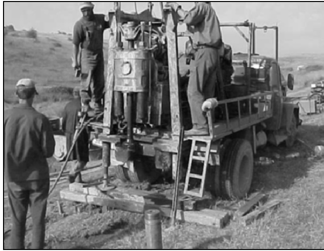
Figure 1. Local contractors in Kosovo drilling a water supply well near Camp Bondsteel. Source: USACE, ERDC, Topographic Engineering Center.
