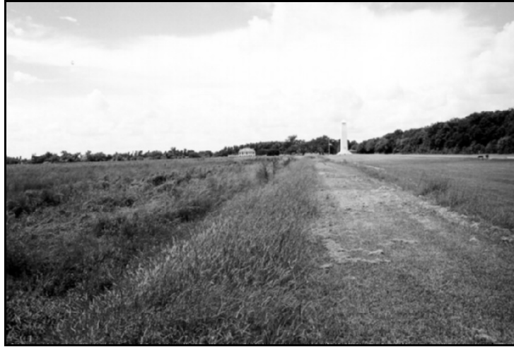
Figure 2. View of Jackson's line looking toward the river along the constructed berm.
