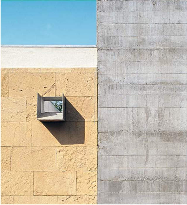
Detail of the wall structures
