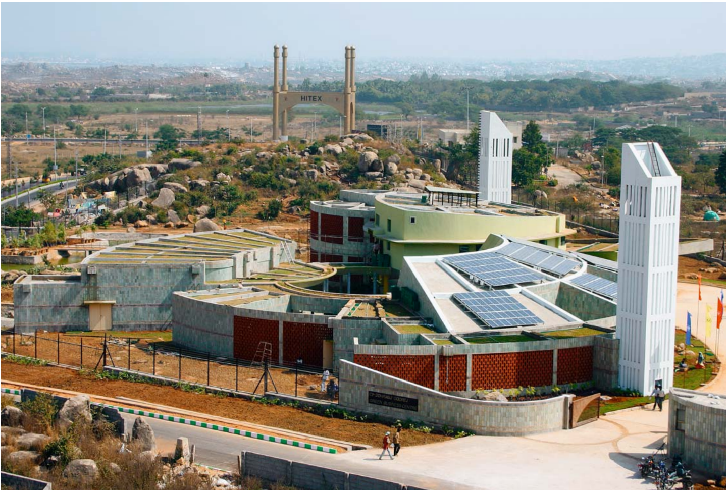
Full view of the complex
