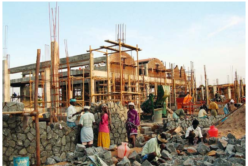
Raising the rubblestone walls
