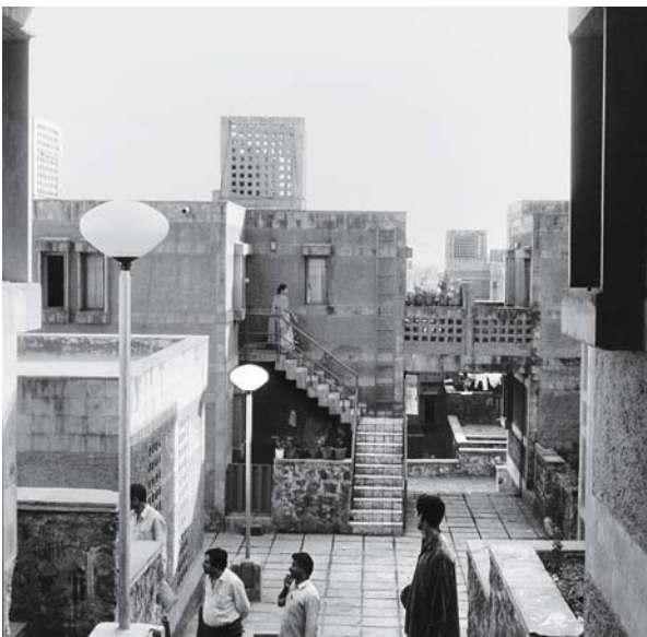
Courtyards and terraces
