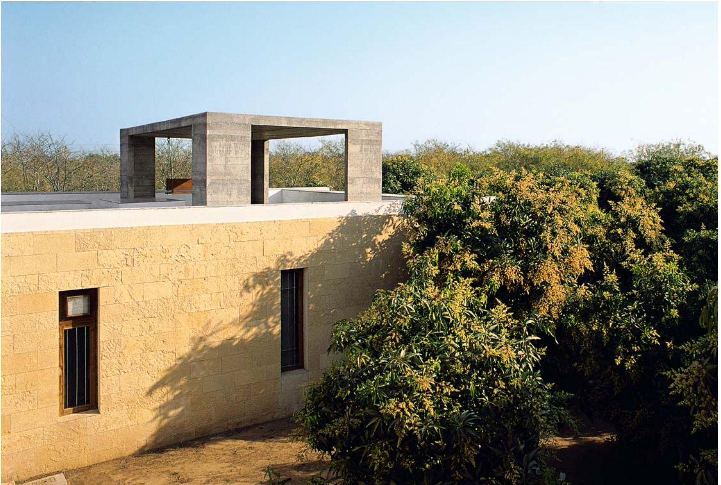
Main entrance — The building in the plantation with pavilion
