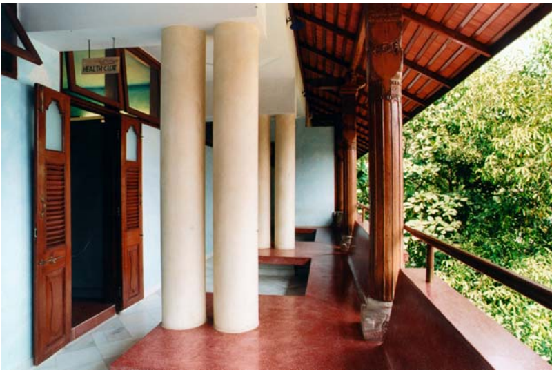
Exit to the third floor roof terrace — The loggia for the second floor waiting area
