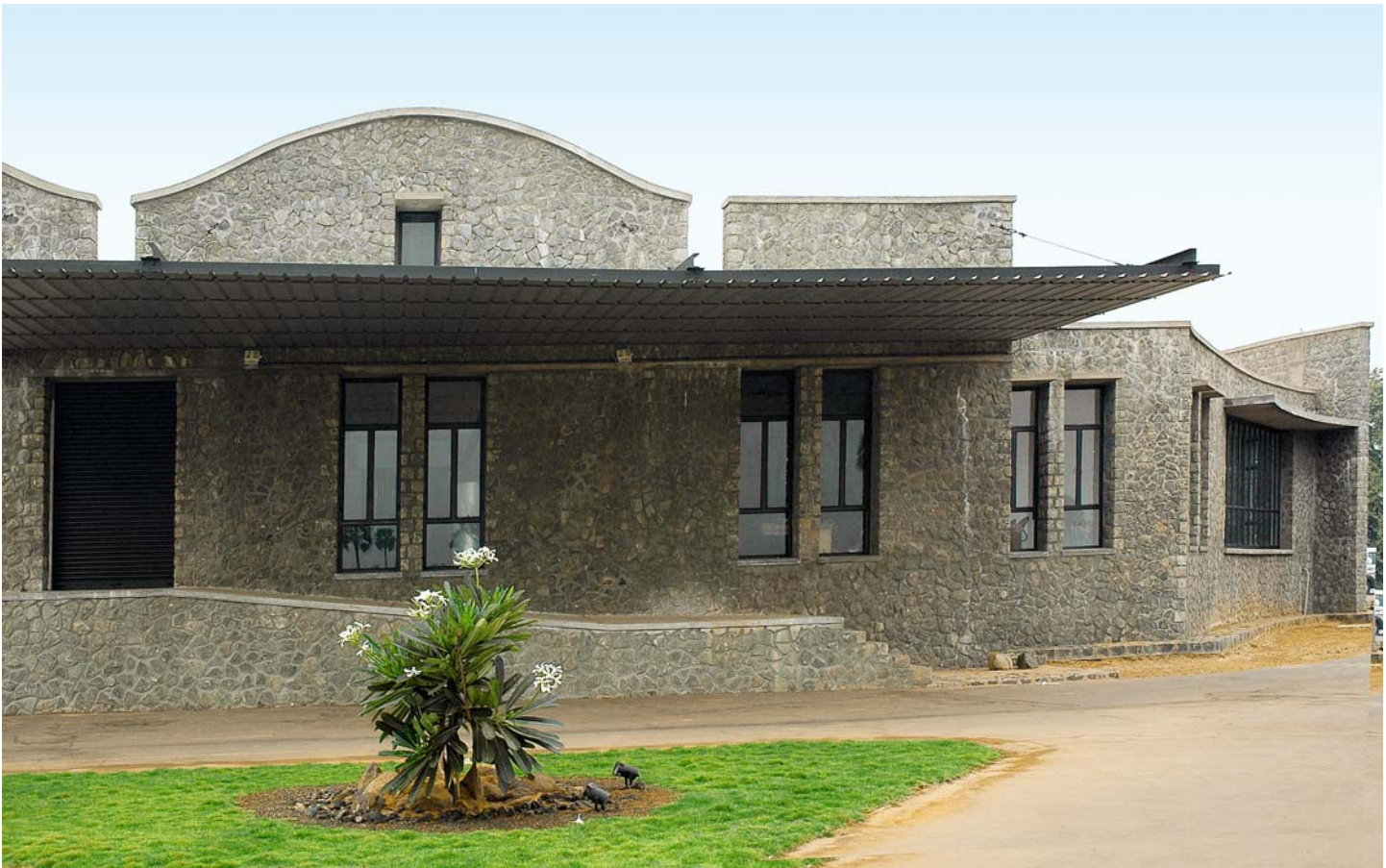
The production area from the rear
