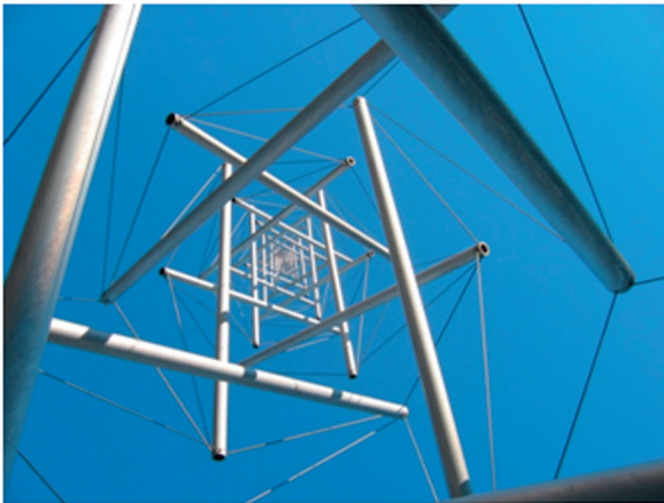
Figure 13.7 Photograph of Kenneth Snelson's Needle Tower (1968), currently housed at the Hirshhorn Museum and Sculpture Garden in Washington, DC. This image illustrates the discontinuous compression member property of tensegrity structures; this property is considered to be the distinguishing and representative feature of a large proportion of Kenneth Snelson's body of work. Illustrating this work contributes to understanding of tensegrity structures and the significance of Snelson's work in twentieth-century sculpture and biology.
