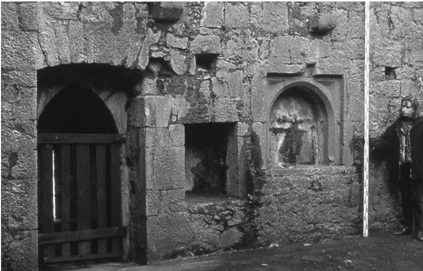
Figure 6. Interior of upper floor of “Fethard Castle” showing entrance doorway from the stair on the left, the spaly of the cross-shaped window in the centre, and the laver on the right.
