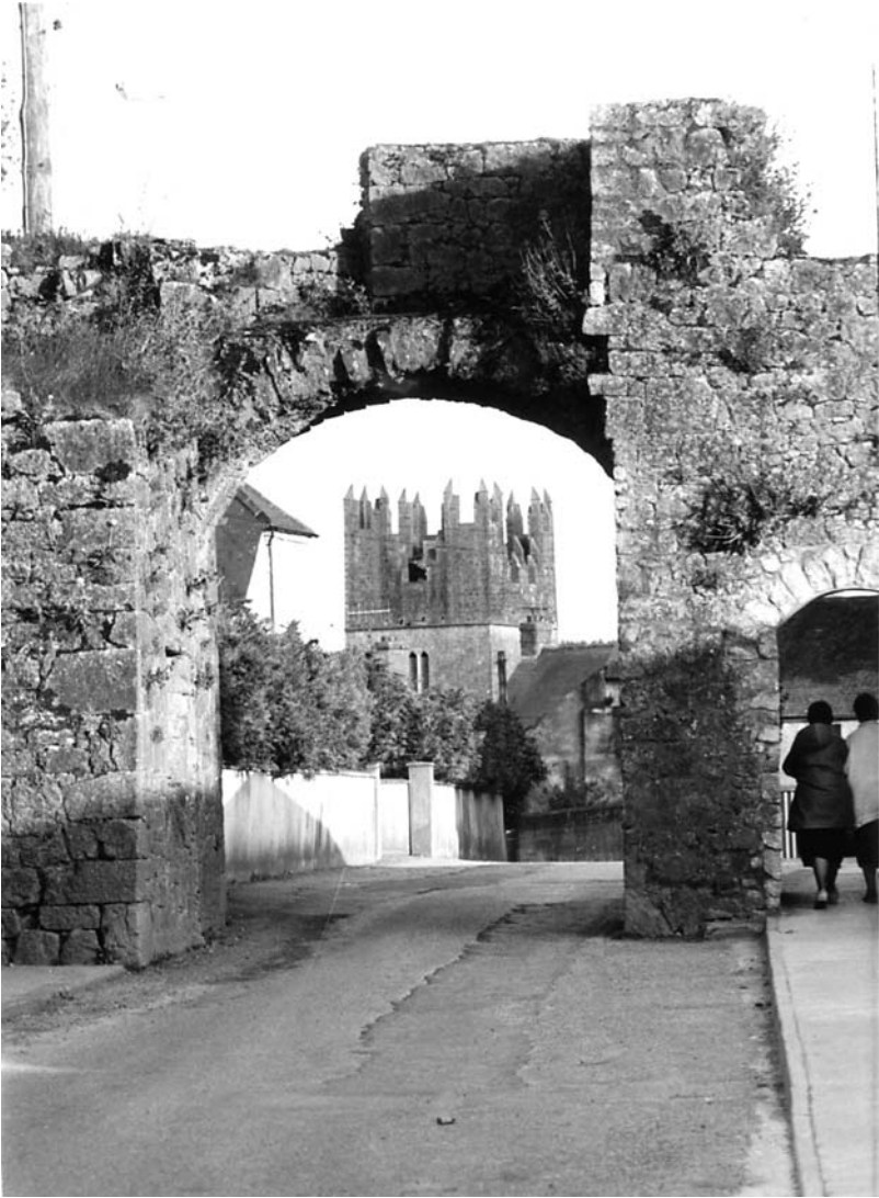
Figure 4. North Gate, the sole surviving town gate in Fethard, viewed from outside the Town Wall; the tower of Holy Trinity medieval parish church is in the background.
