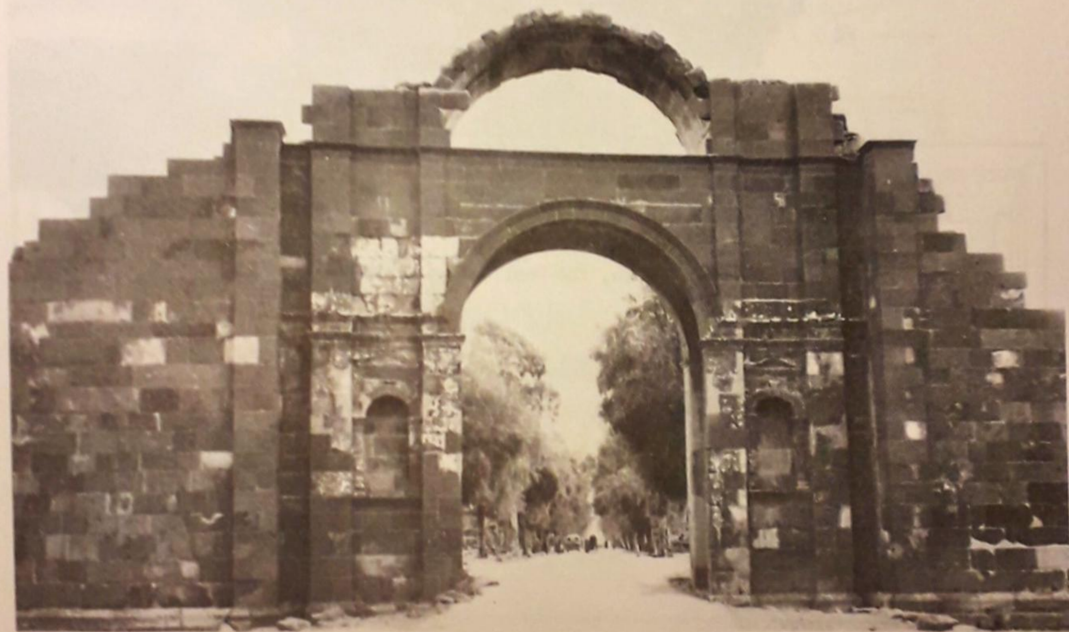
Fig. 117. Bostra, the West Gate, photograph from early 70's.
