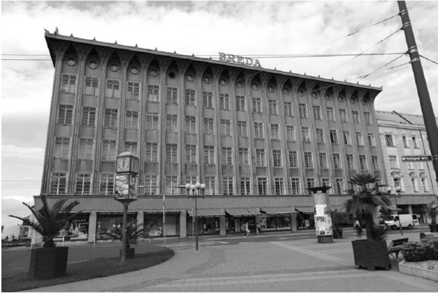
Fig. 8.18 Façade with highly repetitive content. Making close-up photographs from two ends of such building will produce ambiguous result. This is the type of input to be avoided
