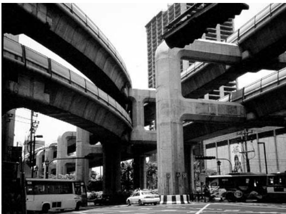
Fig. 3. The massive structure of the Skytrain's line and stations over Bangkok's streets (Source: Mike Jenks)
