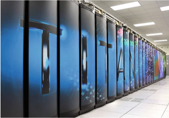
Fig. 2 ORNL's Titan supercomputer, which employs weak parallelism to connect a large number of individual computers for complex problem-solving. This is the most common arrangement for today's high-end scientific systems. Only a small part of Titan, currently the second-fastest computer in the world, is pictured here
