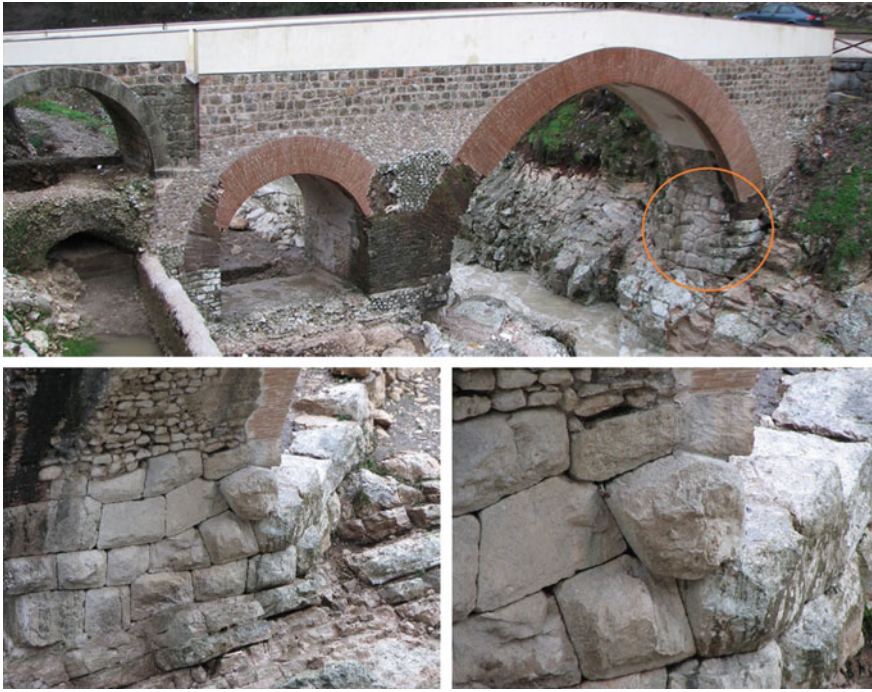
Fig. 22.7 Fabio Massimo Bridge near Faicchio, Benevento, Italy
