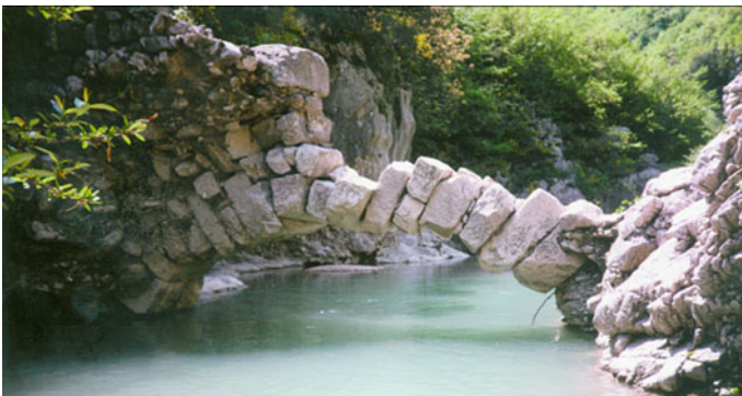
Fig. 22.5 The polygonal construction bridge over the Titerno stream, Italy
