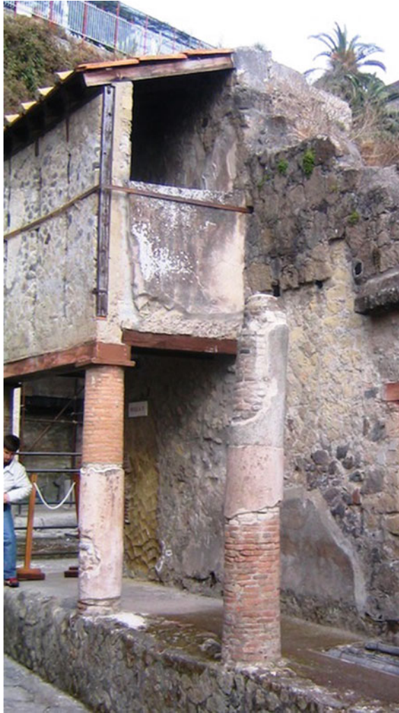
Fig. 22.9 A house in opus craticium in Herculaneum, Naples, Italy
