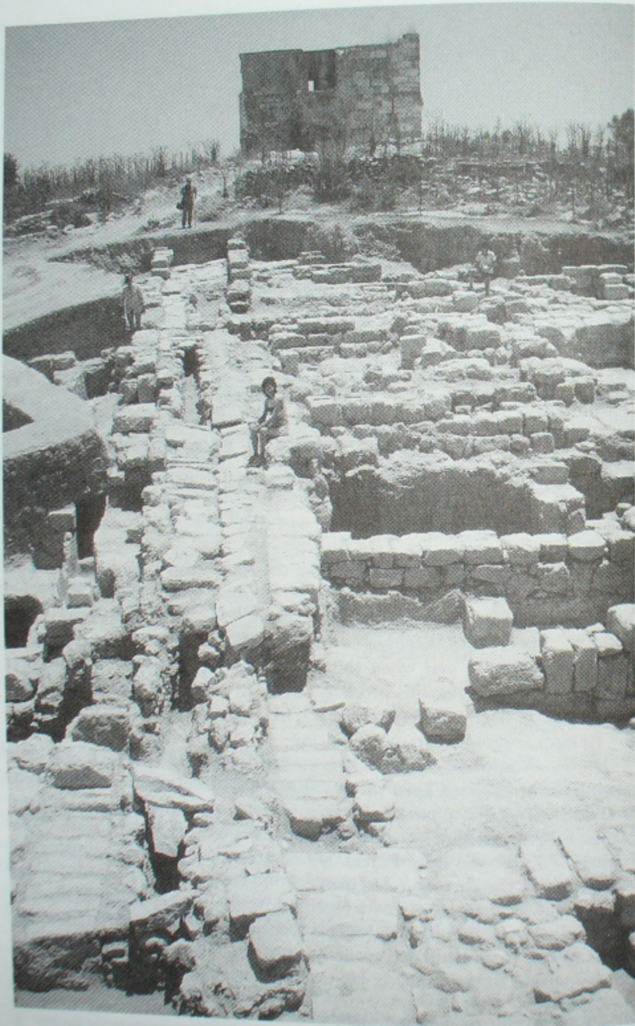
Figure 12.7. East-west roadway with underground drainage visible, western summit.
