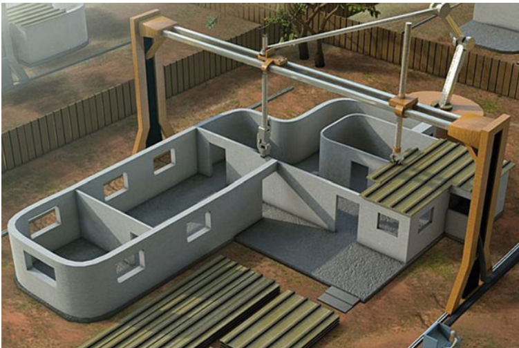
Fig. 4.2 A schematic of an in situ 3D printing of a house. Image Source Flickr
