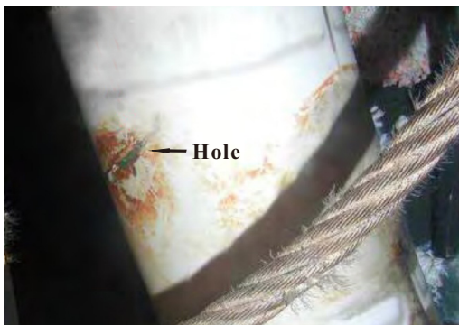
FIGURE 5.7 Hole in the Outer Sheath . Source: Kaye [9]. (For color version of this figure, the reader is referred to the online version of this book.)
