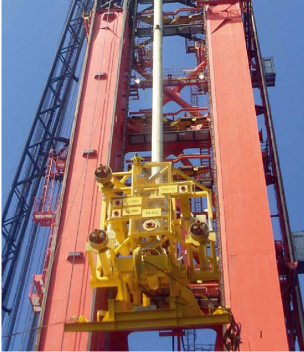
Figure 1-10 Subsea PLET (Courtesy Shell)
