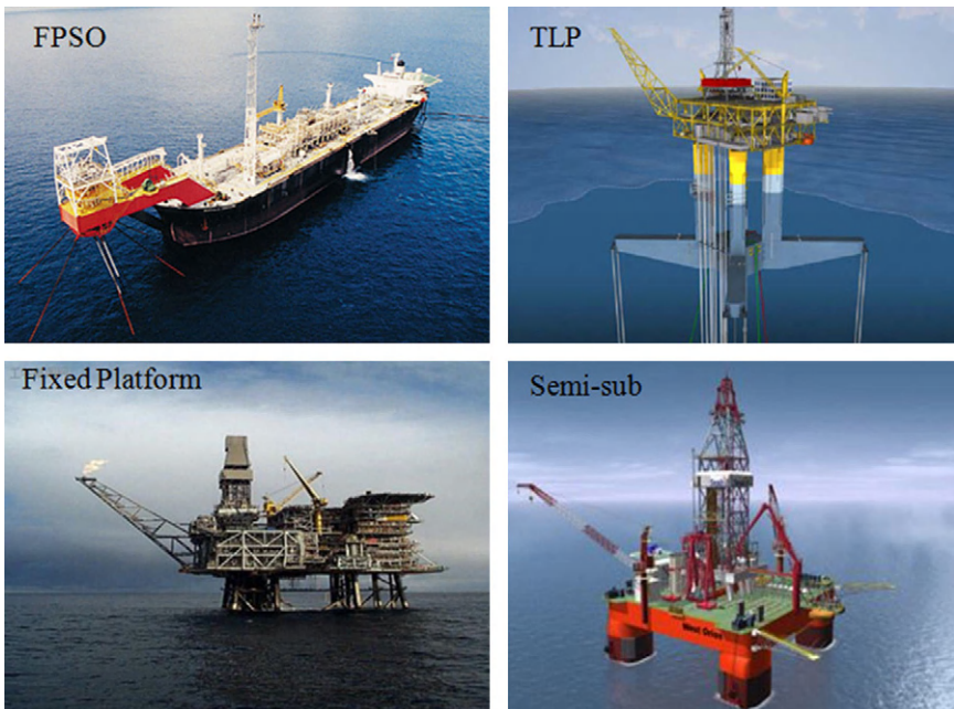
Figure 2-13 Typical Host Facilities
