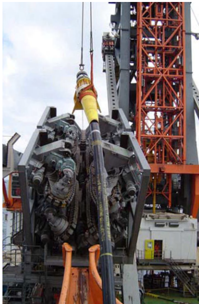
Figure 26-24 Lifting of a Flexible Jumper from a Barge
