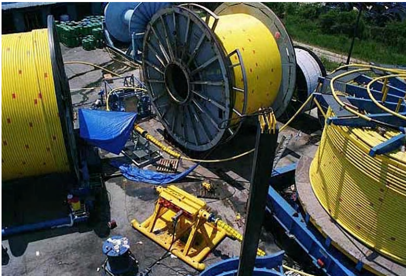
Figure 24-9 System Integration Testing of Control Umbilical
