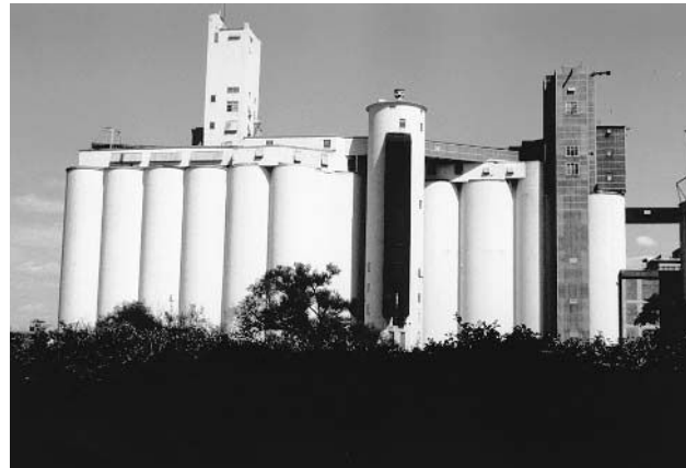
General Mills (formerly Washburn-Crosby) Elevators, Buffalo, New York, 1903 (courtesy Mary Banham)
