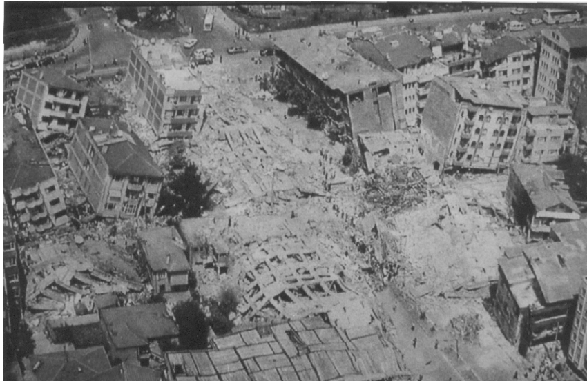
Figure 4: Representative view of a portion of Adapazari that suffered total damage ( I_{EMS-98} = XII ) after the 17 August earthquake.
