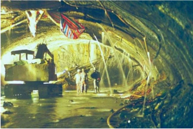
Fig. 1.44 Groundwater affects tunnel construction
