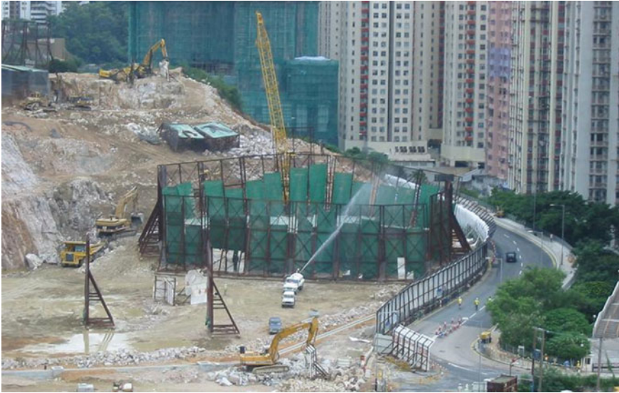
Fig. 11.12 Vertical screens and cages to prevent flyrock
