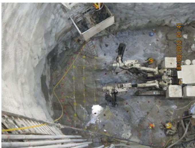
Fig. 16.7 A small two boom jumbos are drilling blastholes in shaft
