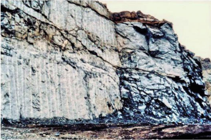
Fig. 10.1 Comparison between the results achieved using control blasting ( on the left ) and normal bulk blasting for a surface excavation in gneiss
