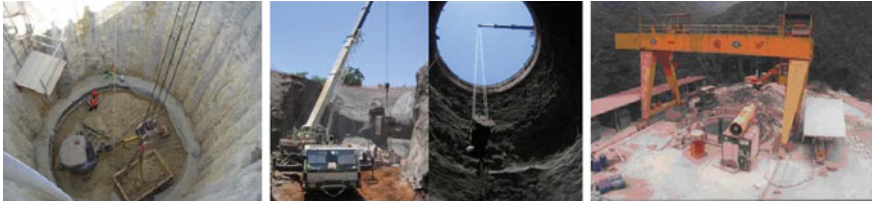
Fig. 19.15 Simple equipment for shallow shaft sinking operation
