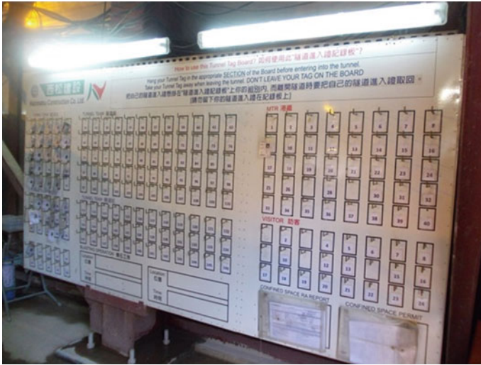
Fig. 23.1 Board of tally system which is located at the entrance of underground construction for check-in and checkout of all personnel
