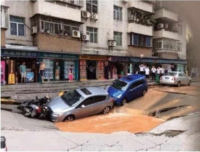
Fig. 23.2 Ground settlement during underground excavation for construction of Metro Line 7 of Shenzhen in June 2015. This accident caused the death of one person and four injured
