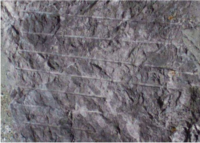
Fig. 17.1. Tunnel rock face formed by smooth blasting
