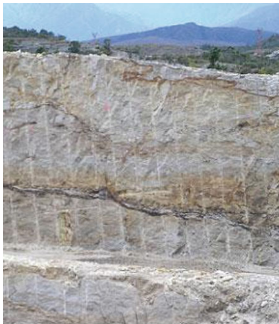
Fig. 10.4 Slope face formed by presplitting
