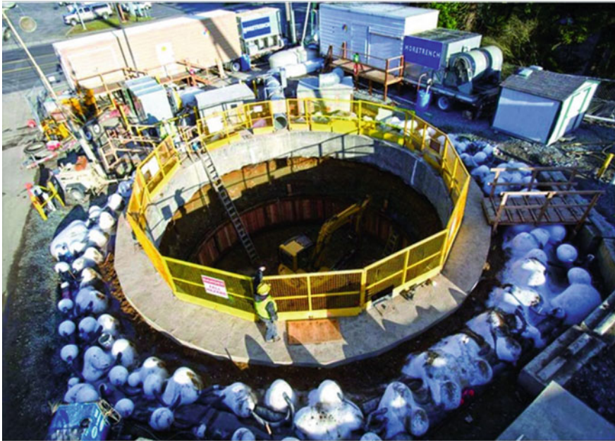
Fig. 21.9 Ground freezing for shaft sinking Source www.moretrench.com/
