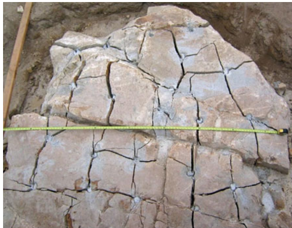
Fig. 7.12 Rock broken by the expansion of cracking agent
