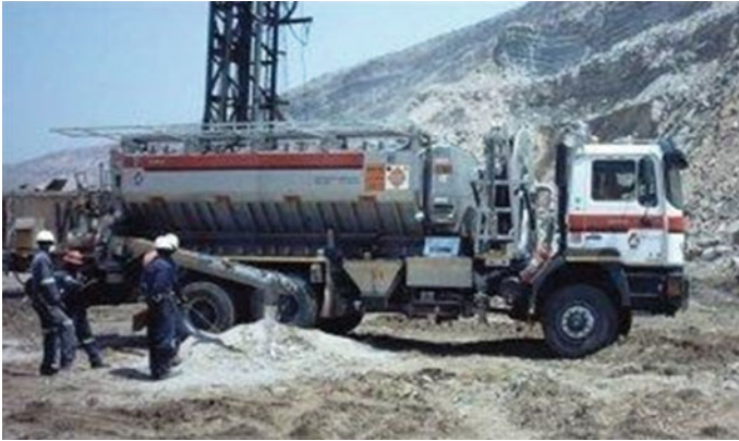
Fig. 3.41 On-site mixing and loading ANFO truck
