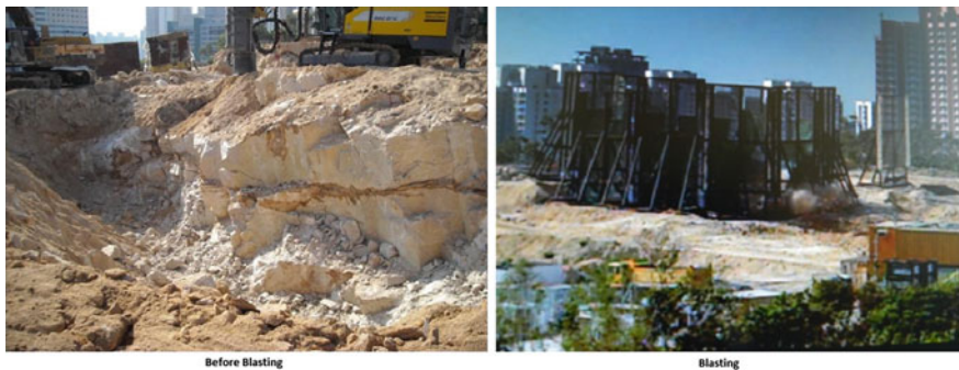
Fig. 1.37 An open joint in rock mass caused high airblast in project DAR, HK, 2009
