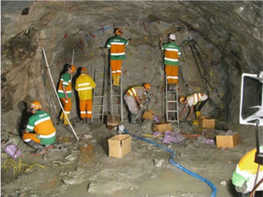
Fig. 16.16 Manual explosive charging in face. Source www.dsd.gov.hk/others/HKWDT/
