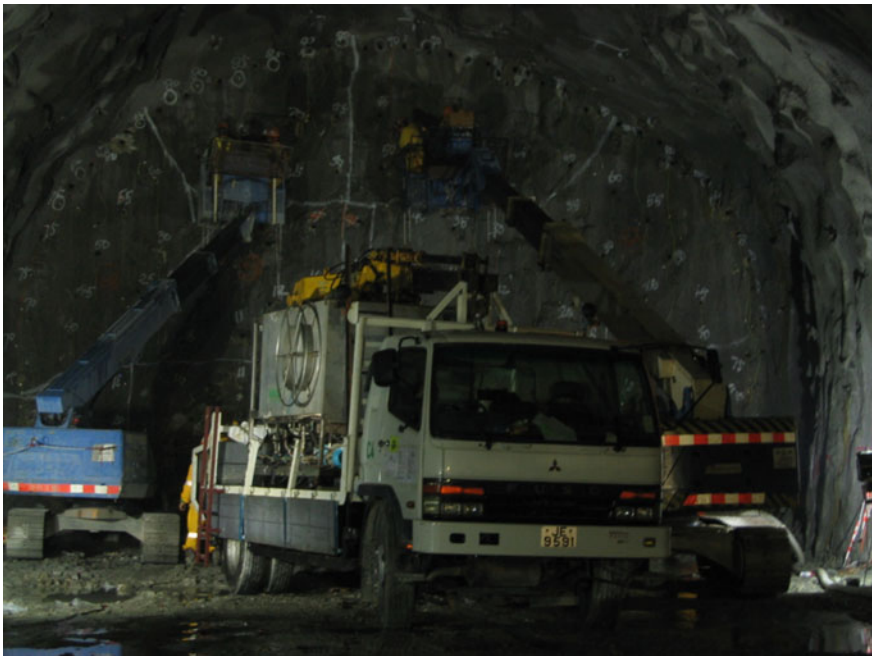
Fig. 16.20 AMSHK’s emulsion pump truck is charging in tunnel face (courtesy of AMSHK)
