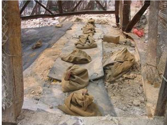
Fig. 11.32 Covering on the presplitting holes
