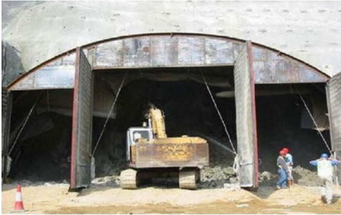
Fig. 23.8 Blasting door for tunnel blasting
