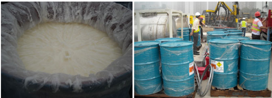
Fig. 3.45 Emulsion matrix was transported to site in drums from factory
