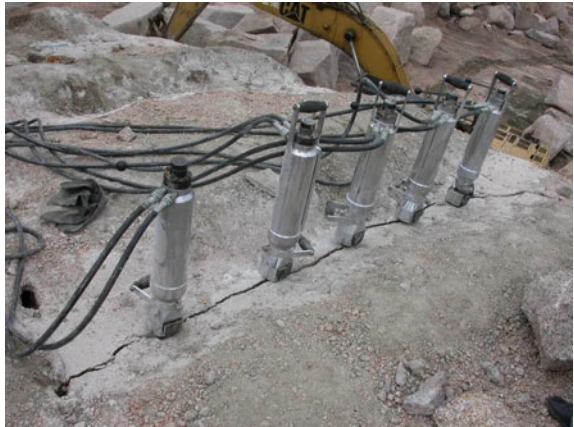
Fig. 7.6 Multi-gun hydraulic rock splitter is working (Courtesy of China Flying Technology Ltd.)
