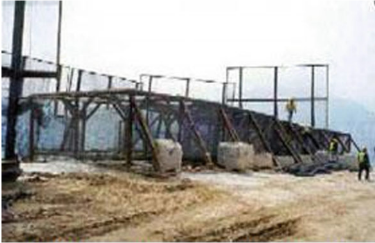
Fig. 11.10 Blasting cages with counterweight
