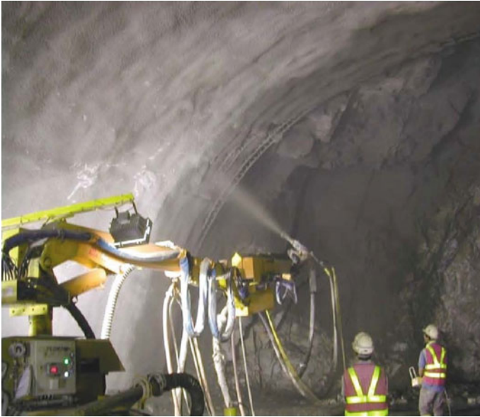
Fig. 21.33 Shotcrete manipulator works in tunnel
