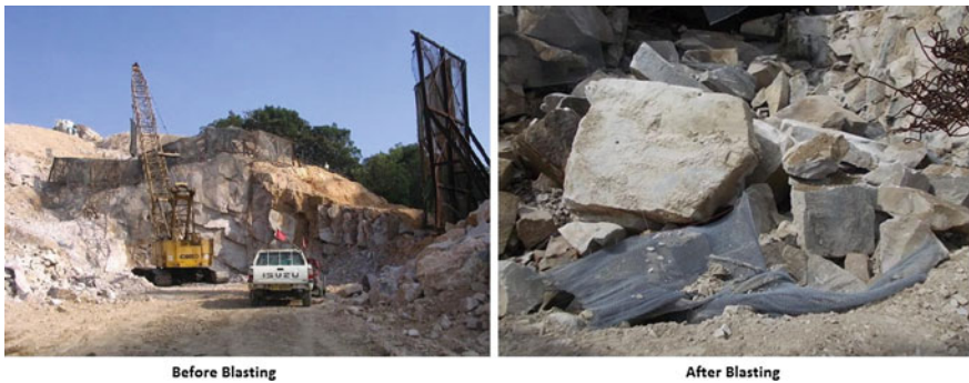
Fig. 1.35 Bad fragmentation by blasting hard and less jointed rock mass
