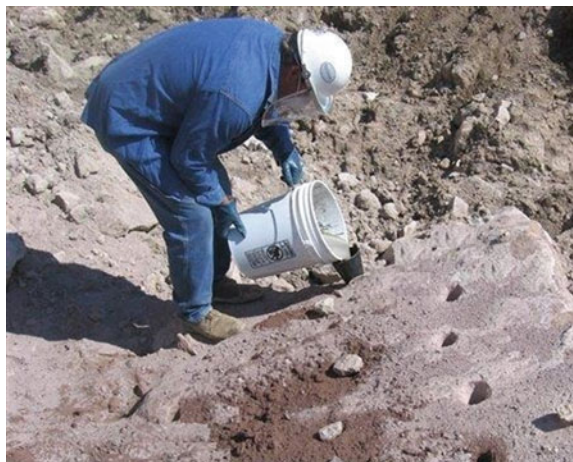
Fig. 7.11 Pouring cracking mortar to drillholes
