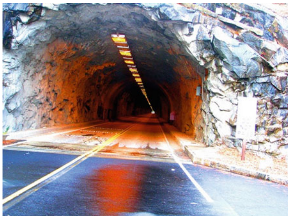
Fig. 21.40 Yosemite tunnel in California, USA, by Rennett Stowe Source www.flickr.com/
