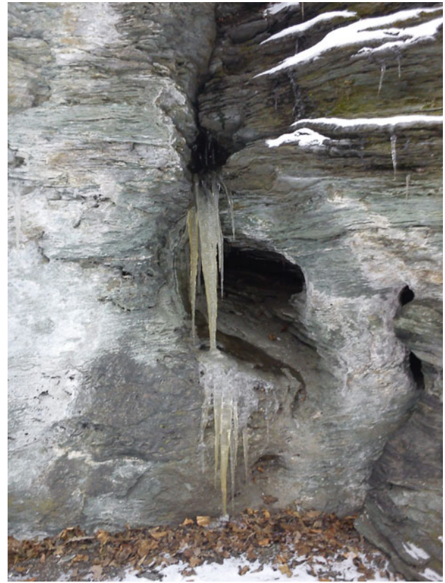
Fig. 6.6 Ice from the niches in greenschists, proving the presence of infiltration and water outflow
