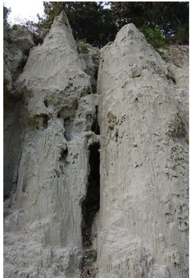
Fig. 18.3 Piping on the wall of Zsidótemplom (photo by Zoltán Karancsi)
