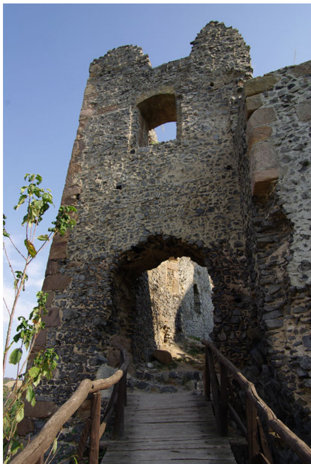
Fig. 17.3 The castle of Somos-kő is built of local basalt columns (photo by Zoltán Karancsi)
