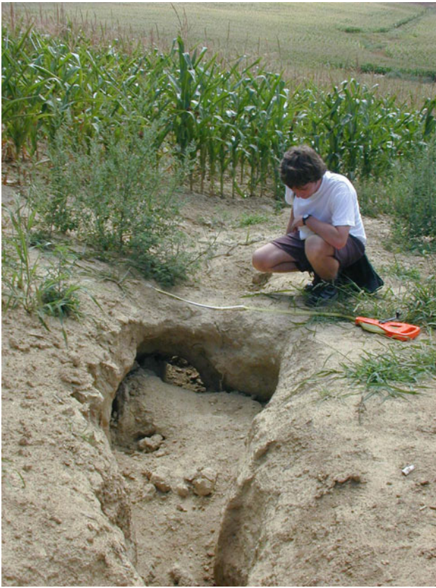
Fig. 12.6 Collapsed tunnel in heavily eroded loess on the border of an intensively tilled arable field. Note the grassed ephemeral gully in maize in the background (photo by Tamás Huszár)
