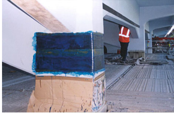
Fig. 11.12 CFRP sheets used in the strengthening of Duarte Pacheco Viaduct
