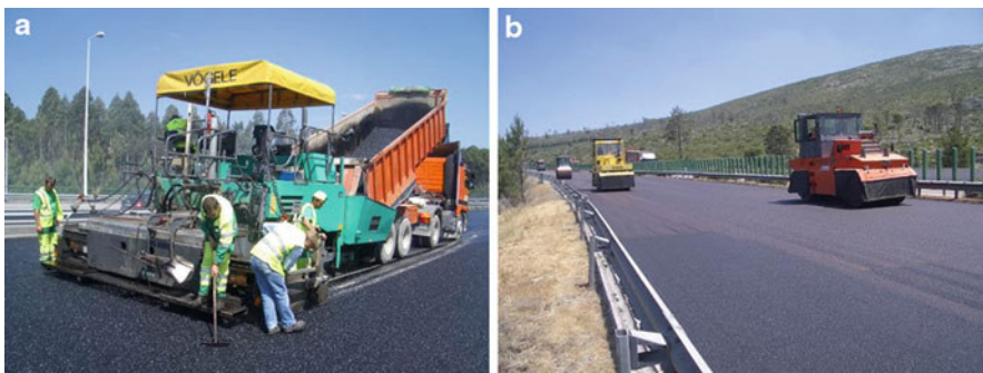
Fig. 5.9 Pavement construction: (a) asphalt paver; (b) rollers operating the bituminous mixture compaction
