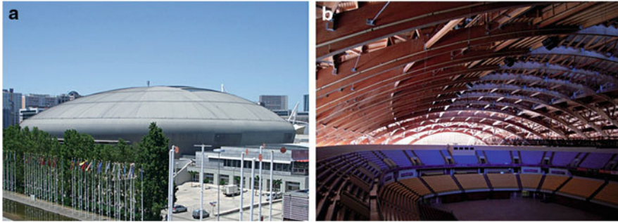
Fig. 16.2 Atlantic Pavilion. The roof structure of the Atlantic Pavilion was the first large glulam structure constructed in Portugal. The structure consists of 17 triangulated transversal arches with variable dimensions, having the largest arch 114 m in length and a maximum height of 47 m above the arena
