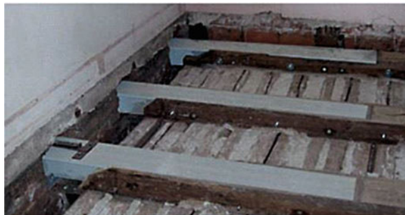
Fig. 11.30 Use of GFRP pultruded profiles in the rehabilitation of a degraded timber floor [32]
