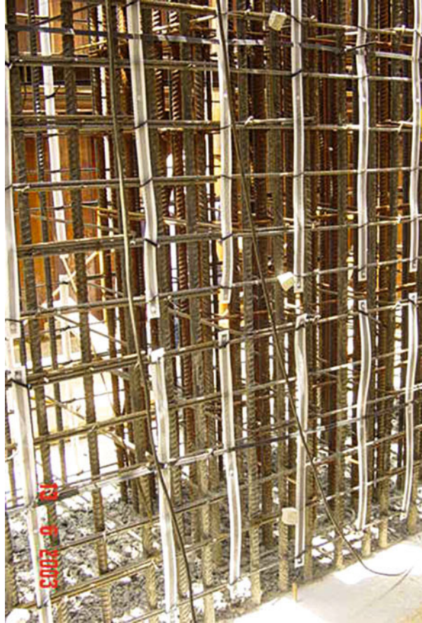
Fig. 15.22 Installation of a cathodic protection system in a structure during construction stage (courtesy of ZetaCorr)
