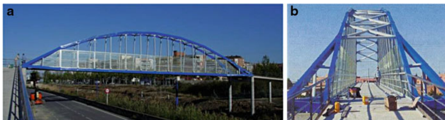
Fig. 11.26 The Lleida bridge: (a) general view (courtesy of Juan Sobrino/PEDELTA) and (b) lateral view [59]
