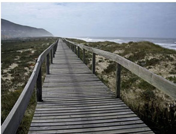
Fig. 12.9 Maritime pine wood showing the typical colour due to weathering
