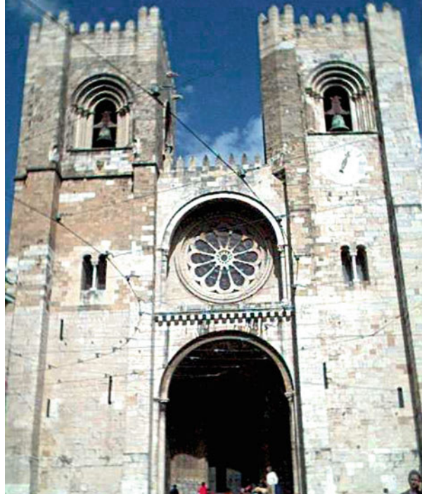
Fig. 15.16 Lisbon Cathedral: aesthetic changes due to air pollution
