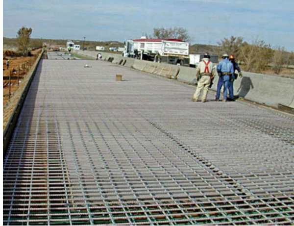
Fig. 11.9 Concrete bridge deck reinforced with GFRP bars
