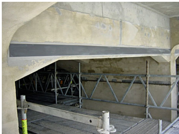
Fig. 11.11 CFRP laminates used in the strengthening of Duarte Pacheco Viaduct
