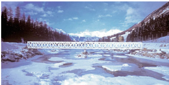
Fig. 11.14 All-FRP Pontresina footbridge [46]
