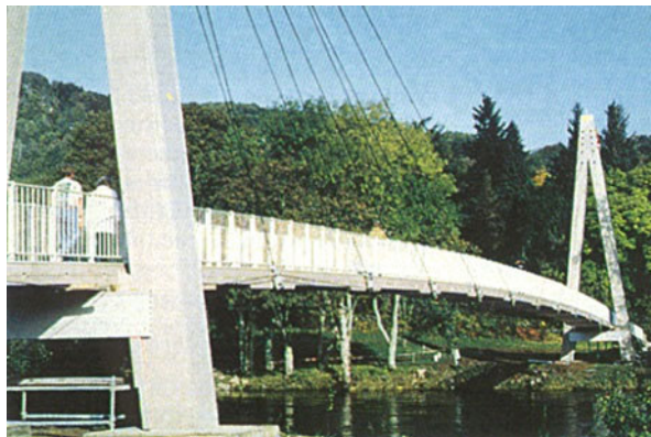
Fig. 11.22 The Aberfeldy bridge [13]
