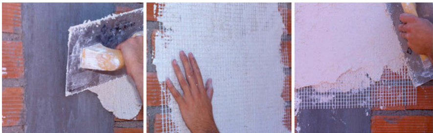
Fig. 2.18 Application sequence of a glass fibre net in the transition zone between a concrete column and a brick masonry wall [64]
