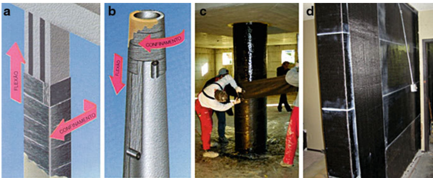
Fig. 11.38 Flexural and axial (confinement) strengthening of (a) columns and (b) chimneys with strips and sheets; use of sheets in (c) columns and (d) walls (adapted from [55, 10, 35])
