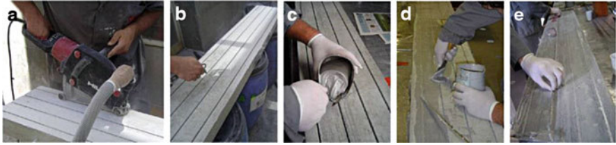
Fig. 11.40 Different stages of the application of a precured FRP system in the strengthening of a reinforced concrete element, according to the NSM technique [11]. (a) Execution of grooves cut onto the concrete cover; (b) cleaning of the groove; (c) mixing the adhesive; (d) filling the groove with the adhesive; (e) introduction of the FRP laminate into the groove
