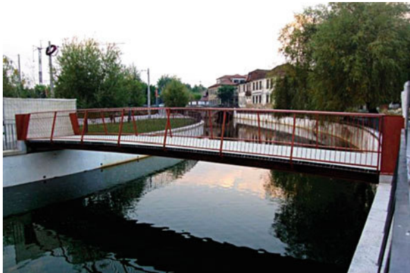
Fig. 11.13 Steel/GFRP hybrid footbridge in Viseu, Portugal
