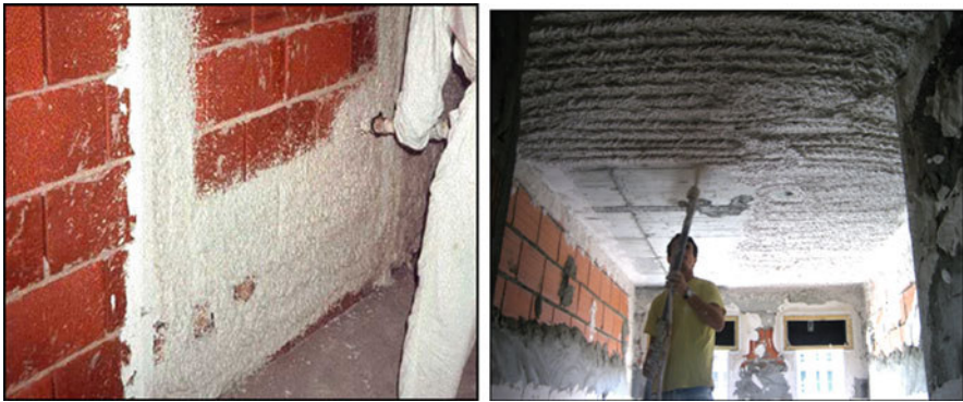
Fig. 3.48 Examples of coating application using spraying devices [27]
