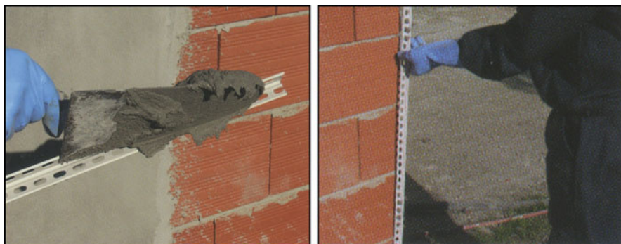
Fig. 3.39 Application of a perforated PVC protection profile in a salient corner of a wall [35]
