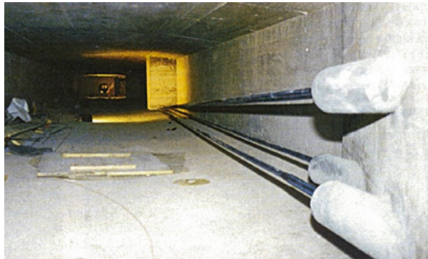
Fig. 11.10 CFRP cables used in external prestressing of Verdasio Bridge [46]
