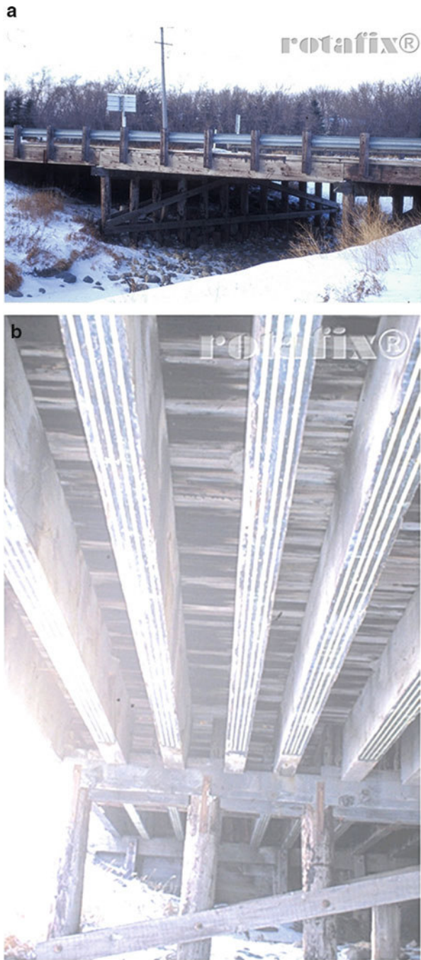
Fig. 16.3 Use of structural adhesives in the repair and strengthening of timber structures (the images were kindly provided by Rotafix Ltd., more information concerning the work illustrated in the figures can be found in [5])
