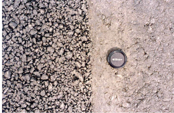
Fig. 5.7 Texture of the pavement surface in porous asphalt ( left ) and asphalt concrete ( right )
