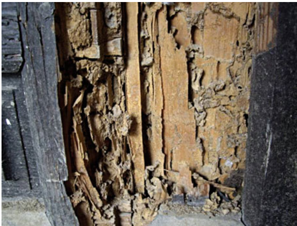
Fig. 12.11 Laminated appearance of the wood and the presence of mud tunnels resulting from the action of subterranean termites
