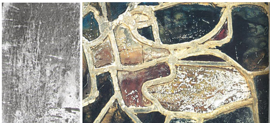
Fig. 8.22 Secondary corrosion: risks and stings in a mediaeval glass from Mosteiro da Batalha (Courtesy of Dr. Pedro Redol, Director of Mosteiro da Batalha, Portugal)
