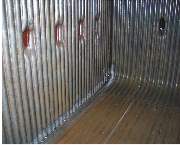
Figure 7.1 Modern furnace walls with air ports.
