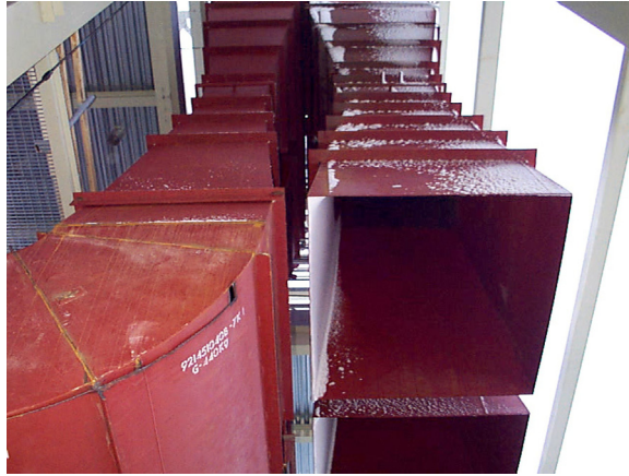
Figure 7.8 Air ducts during construction.
