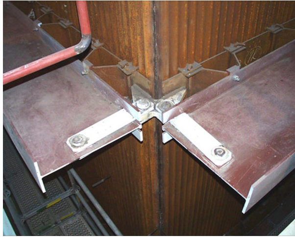
Figure 13.4 Support steel for the furnace wall.
