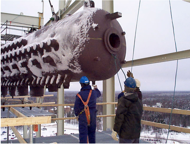
Figure 4.15 Erection of steam drum under wintery conditions.
