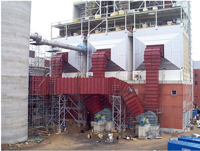
Figure 6.10 Electrostatic precipitator being erected.
