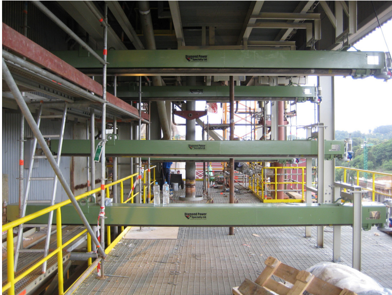
Figure 6.8 Retractable sootblower.
