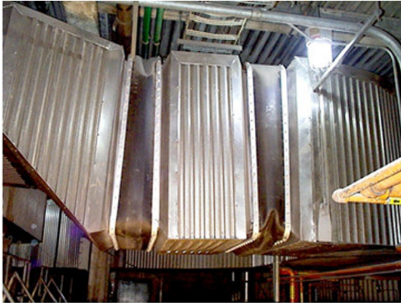
Figure 7.9 Expansion joints in an air duct.
