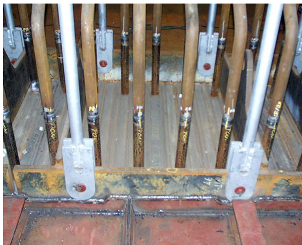
Figure 13.8 Hanging of cold surfaces.
