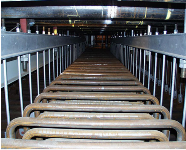
Figure 13.6 Superheater support structure.
