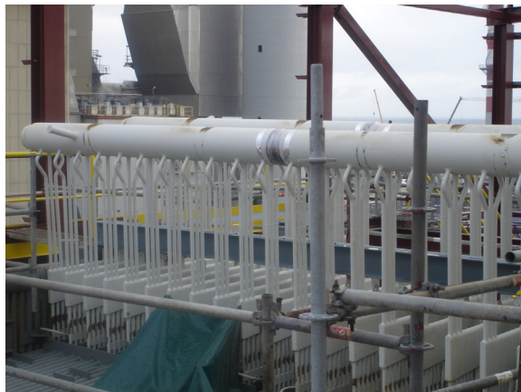
Figure 7.4 Superheaters under construction. Courtesy of Andritz.
