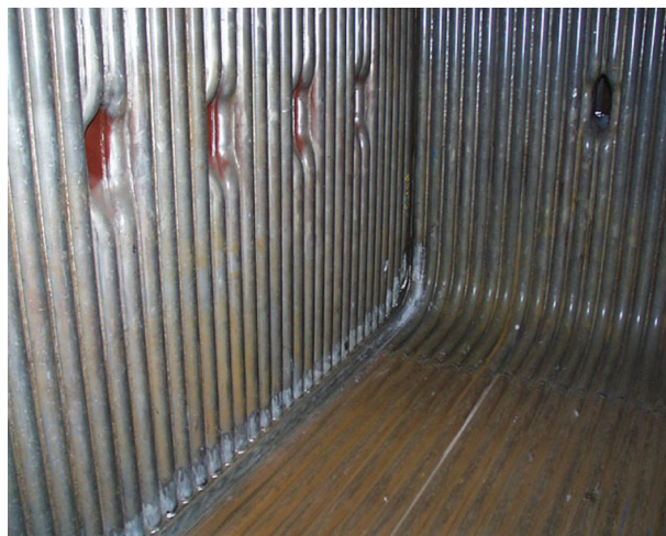
Figure 11.9 Modern carbon steel furnace bottom. Courtesy of Andritz.
