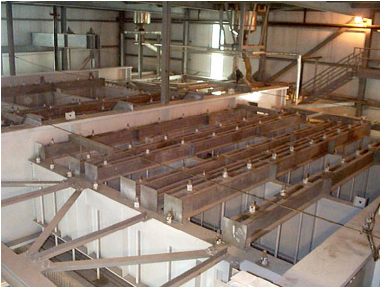
Figure 13.3 Top support beam arrangement.
