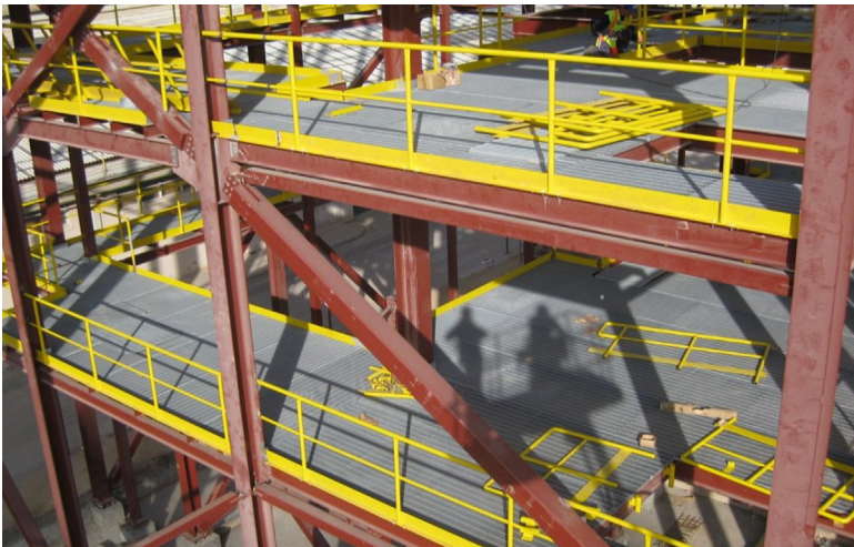
Figure 13.10 Platforms under construction.
