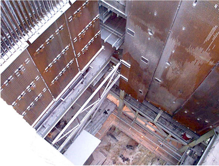
Figure 13.9 Installation of a furnace wall.
