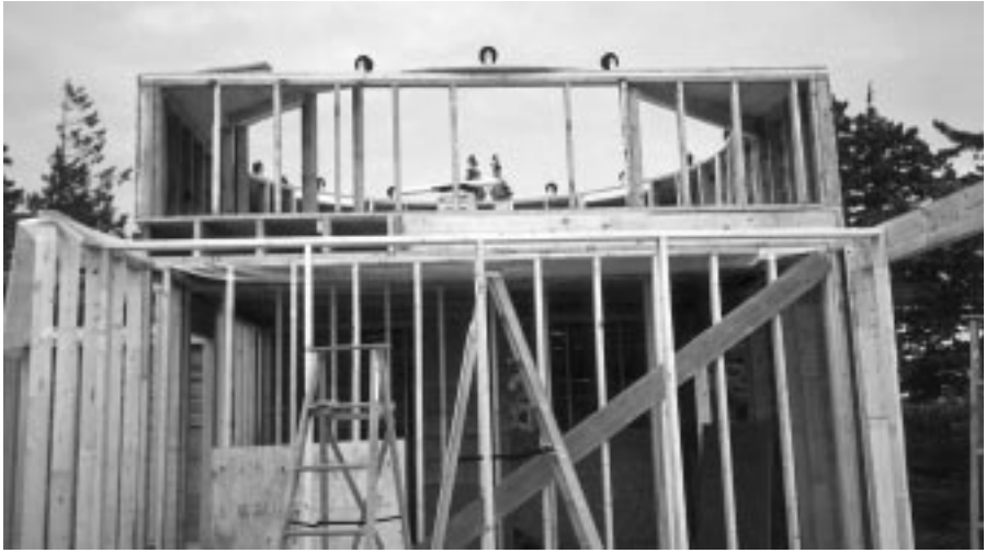
Figure 16.7 The concrete telescope pier (just visible, left of centre) rises through three floors of the house.
