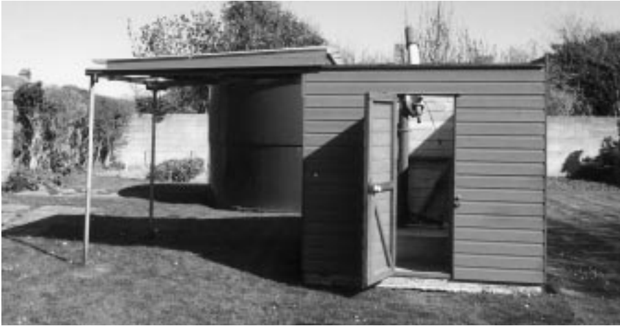
Figure 15.4 The run-off roof shed with its roof slid back.
