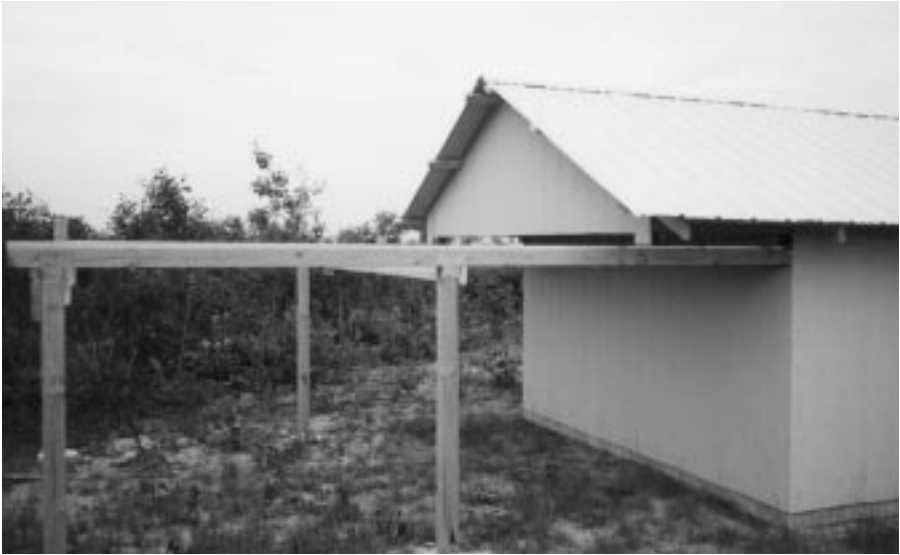
Figure 1.7 External rails with the roof partly rolled.
