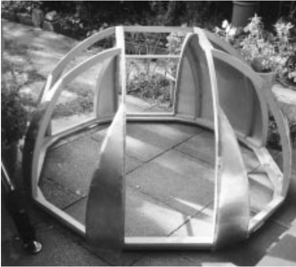
Figure 6.2 The 1.7 m Meade dome; the 16-sided plywood frame is clad in sheet aluminium.
