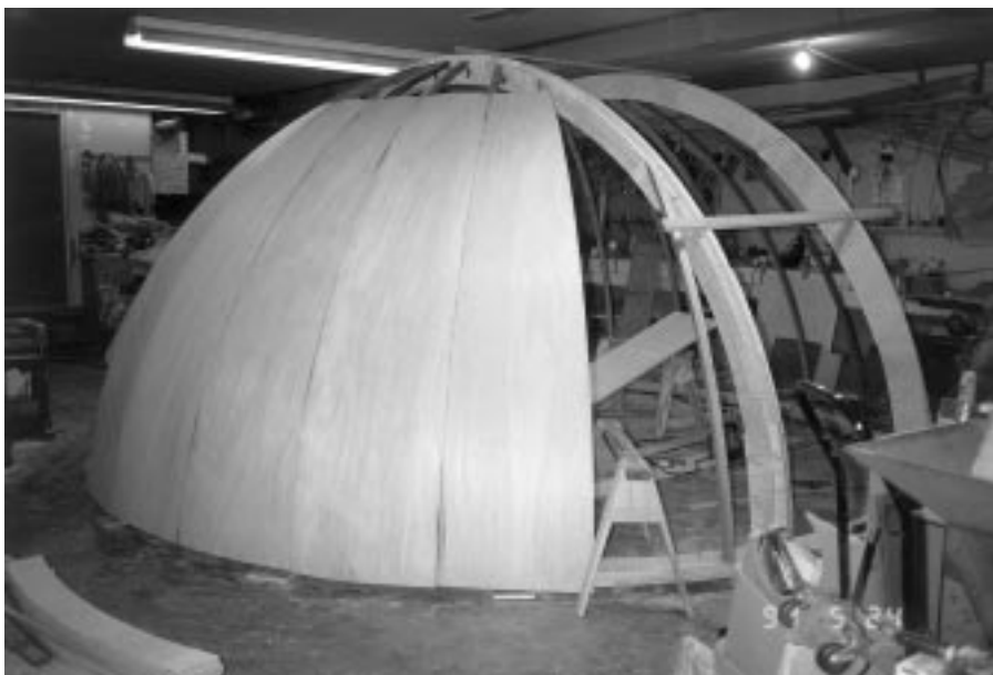
Figure 16.3 The mahogany sheathing seen from the outside.
