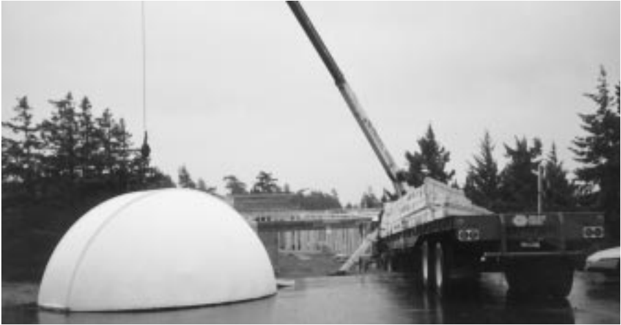
Figure 16.4 The dome about to be hoisted into position on the roof.
