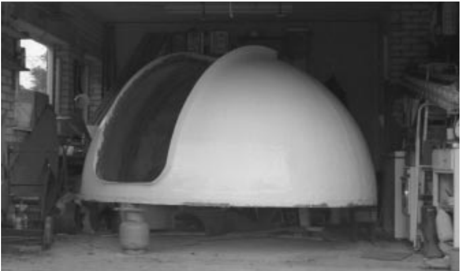
Figure 23.5 The completed dome, with upstand round the slot and fibreglass/resin finish.
