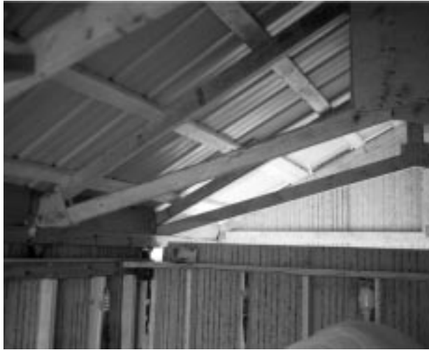
Figure 1.8 The church trusses supporting the roof.
