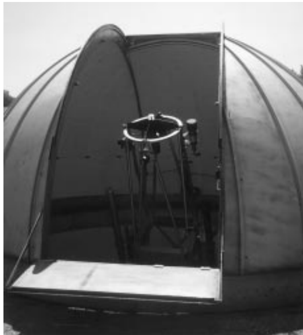
Figure 14.5 The open dome, with polystyrene tiles covering its interior surface.
