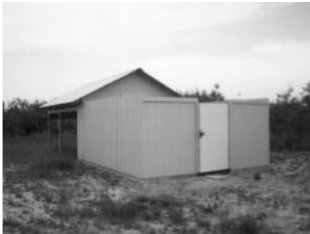
Figure 1.9 The observatory with the roof fully rolled back.
