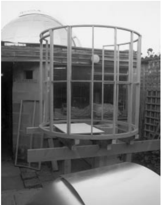
Figure 6.6 a The Meade mini-observatory is supported off two posts and the wall of the main observatory. The left-hand window becomes the observation panel separating the two observatories. b The Meade observatory takes shape.
