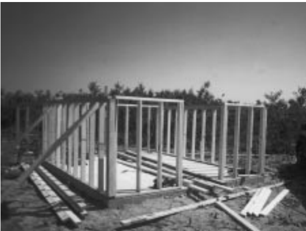
Figure 1.3 Construction of the walls and rails.
