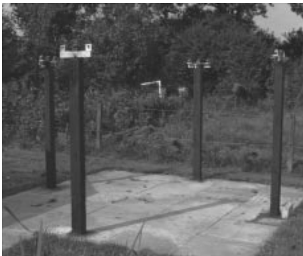
Figure 23.6 The four posts on which the dome rests, each topped with a wheel assembly.
