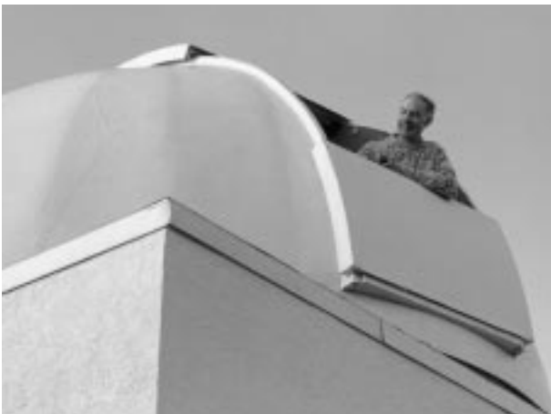
Figure 16.5 The dome-slit, with lower flap and sliding upper section.
