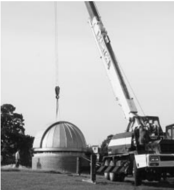
Figure 14.2 The dome being lowered into position.
