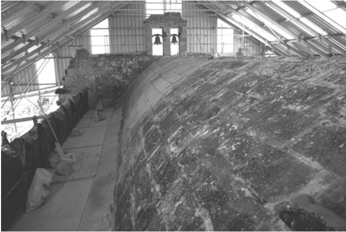
Fig. 15 View of the enclosed church roof of Rosslyn Chapel just before the refurbishment measure
