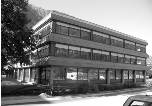
Fig. 9 Zams-Schönwies the south façade before renovation. Photo Robert Ehrlich
