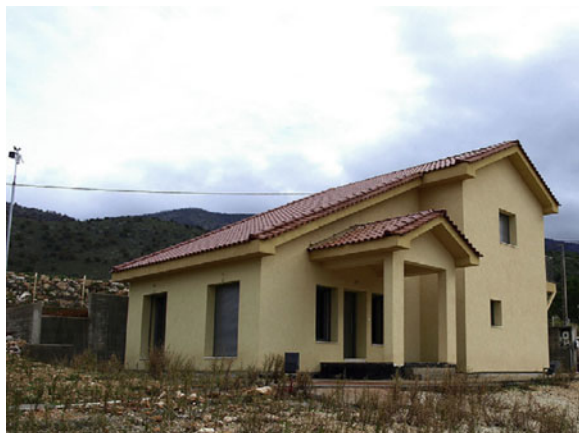
Fig. 4 External view of a demo house including PCM wallboards (Mandilaras et al. 2013)
