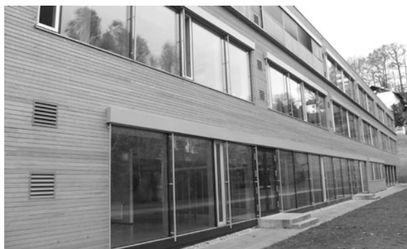
Fig. 2 Schwanenstadt: a compact shape and large windows for increased daylight. Shading is provided by venetian blinds. Square vents for the decentralised ventilation units are visible. Photo Xavier Dequaire
