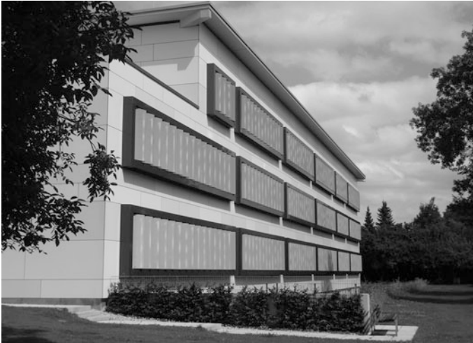
Fig. 20 View of a refurbished school using VIP for the insulation of the base slab
