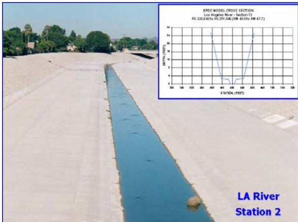
Figure 6. Channel Cross-Section at LA River Station 2
