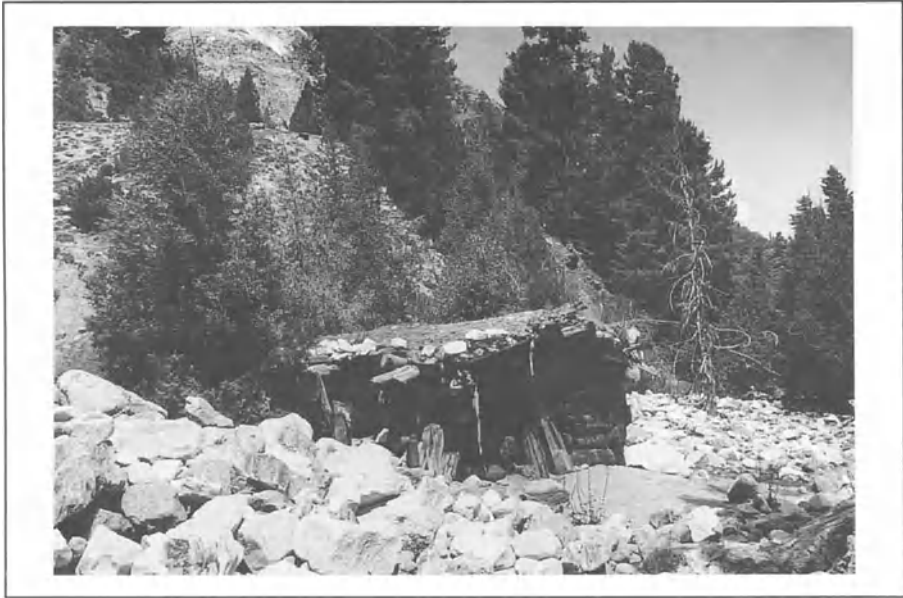
Figure 11. Remaining building at edge of Biale village partly buried by the south Biale debris flow of 1990 in the Raikot valley of Nanga Parbat. This building was not overwhelmed but boulders were piled up around it.
