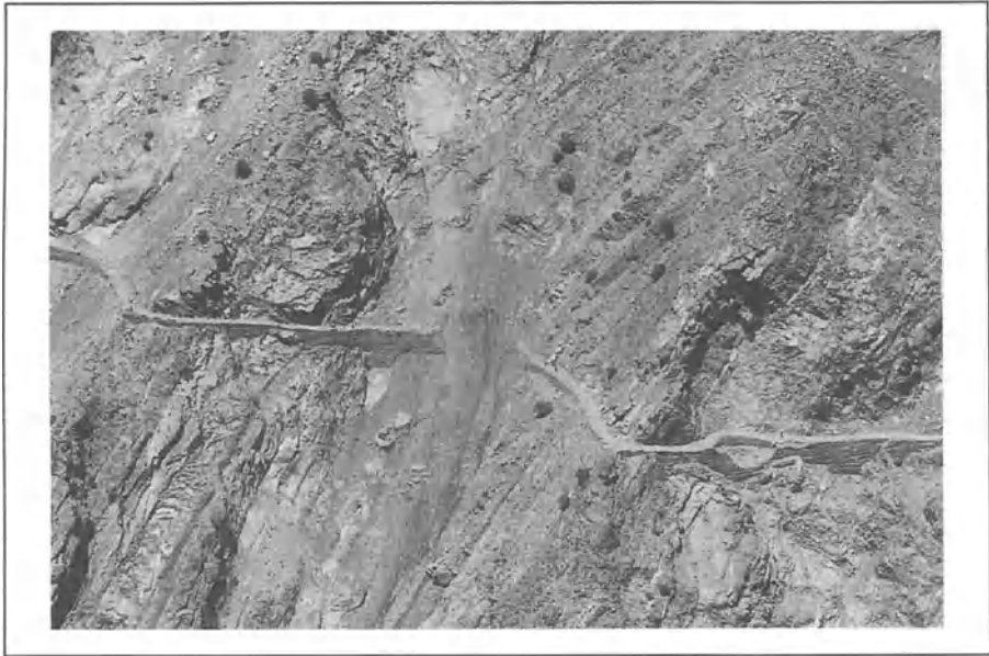
Figure 13. View down on the Tato road from the KKH up to Raikot basin in summer 1996 showing slope failure being crossed by villagers on foot. The road was out of use to wheeled traffic all summer during the high traffic tourist season upon which the villagers depend as their only source of income in a subsistence economy. Such natural hazards are extremely common on the steep slopes that are characteristic of the Himalaya.
