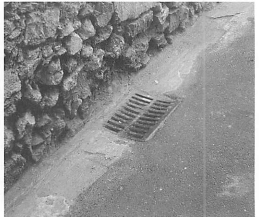
Ravello: Ordinary gutter and drain—just right
