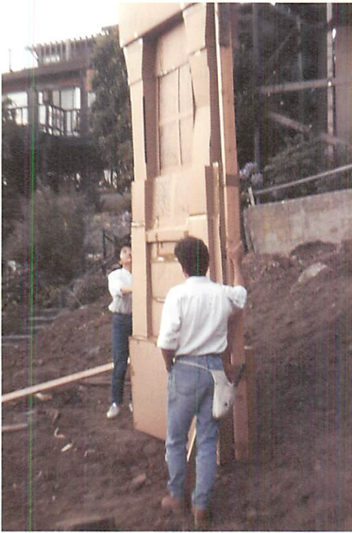
Looking at the cardboard mockup on the site, to test its feeling in relation to the site
