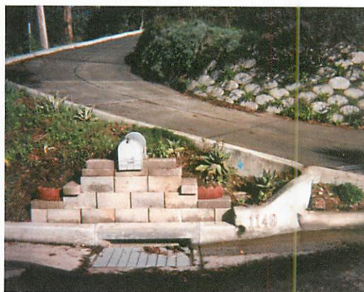
Mailbox which is not structure-preserving. The center which is created under the mailbox does not arise naturally from the surrounding wholeness.
