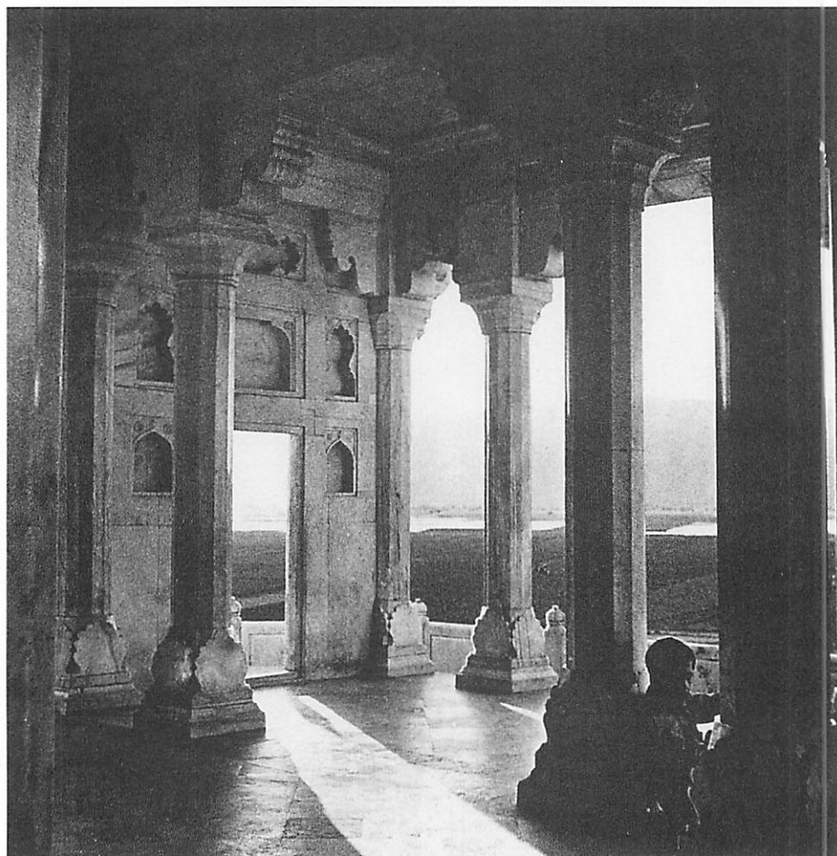
The love of the distant mountains makes it possible to build this porch, with its tall columns, as an extension of the mountain land
