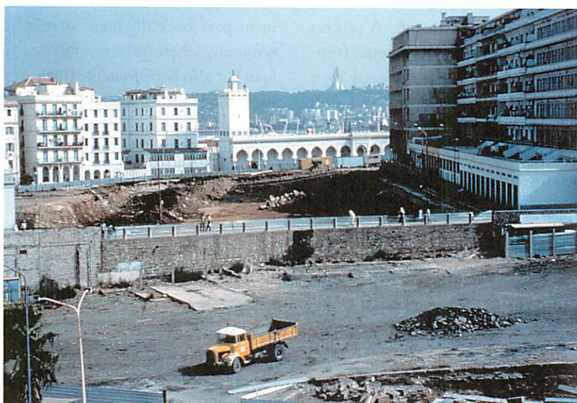
The beginning of the slash: preparation for high construction destroys Algiers.
