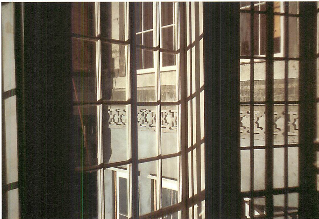
Close-up of living room windows after installation
