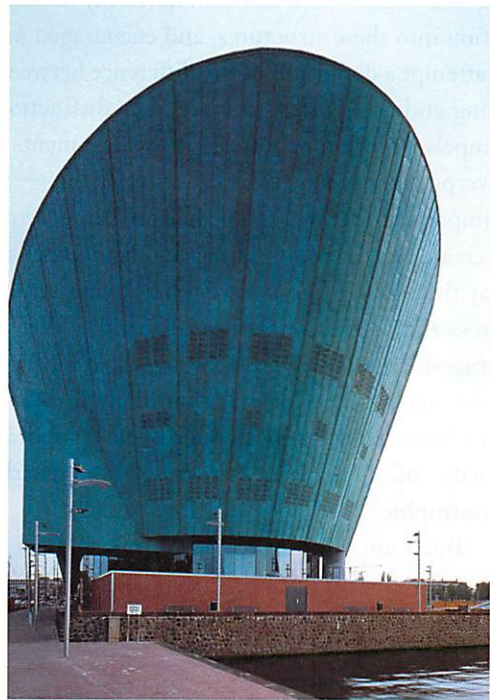
Non-living structure: Technology center, Amsterdam
