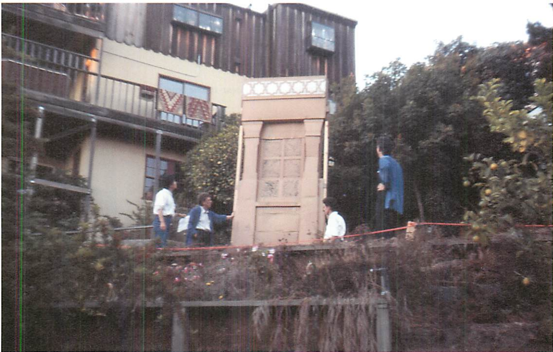
Cardboard mockup of wall construction. This mockup was very detailed, full size, and allowed us to check the offset between one plane and another to the nearest half inch and quarter inch
