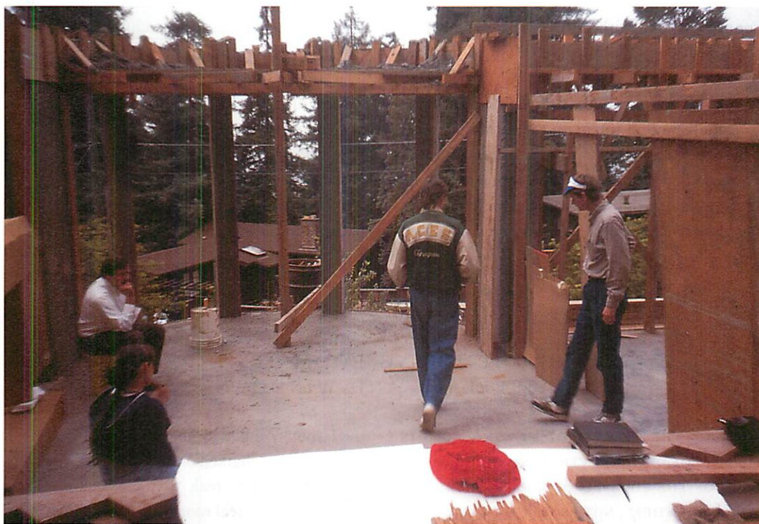
Walking into the room, testing the position of the door, and trying to find out if the positive space of the bay window is large enough, when the door is in a certain position. We moved this door several times, and finally tuned it to within about two inches to get its best position.
