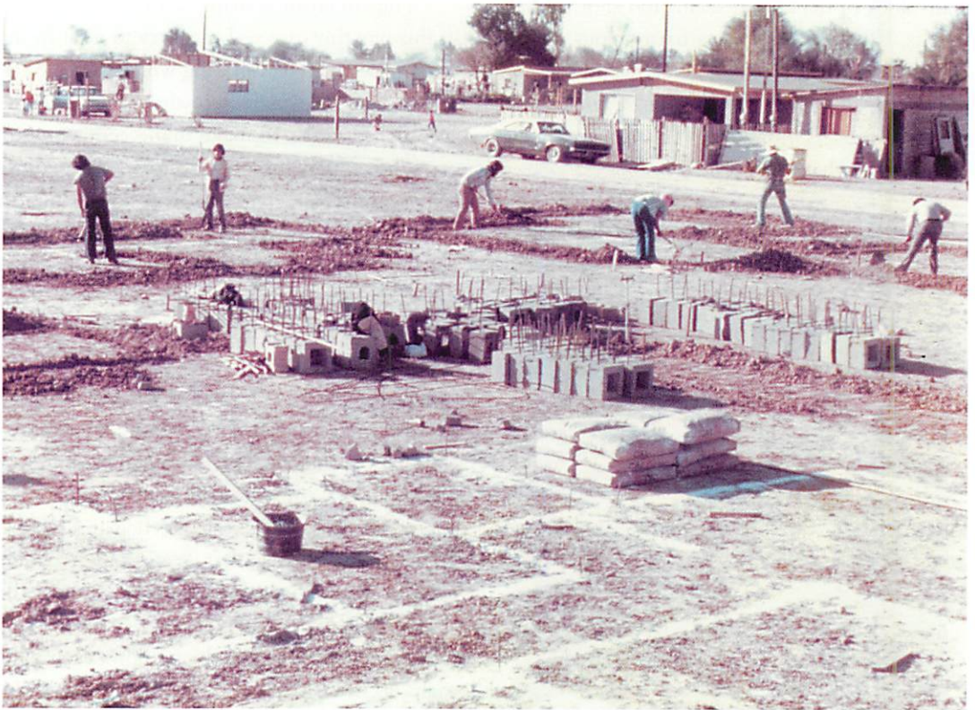
Forming centers in the early stages of a house-building process in Mexico. From the very start, the emphasis is on step-by-step adaptation: design and construction are integrated. Christopher Alexander, Julio Martinez, Howard Davis, and others, Mexicali, 1976.
