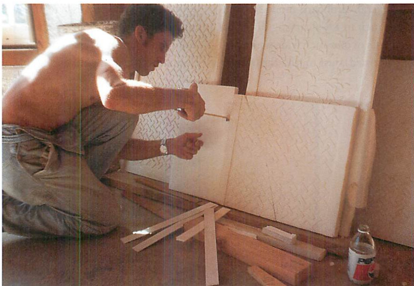
Randy checking widths and details of the edge band on the plaster panels. On these panels, it turned out that a difference among one-eighth, one-quarter, and three-eighths of an inch was of tremendous significance.
