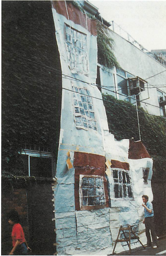
Emoto Apartment Building, Komagome, Tokyo, Christopher Alexander, Hajo Neis, Ingrid King, 1987. This full-size three-story mockup in Tokyo, done in paper to study the effect of the elevation design and materials on the street at actual size, was done to make sure that the street was helped by the building. Mockup by Hajo Neis.
