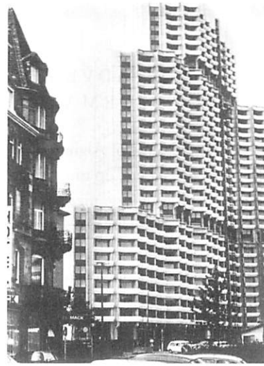
The highly repetitive structural scheme makes no adaptation to the location of the structural bays, or to relative closeness to the ground. A structure-preserving process would reflect the structure at each place in the building, as a function of the position and condition of that particular place, thus creating an organic structure.
