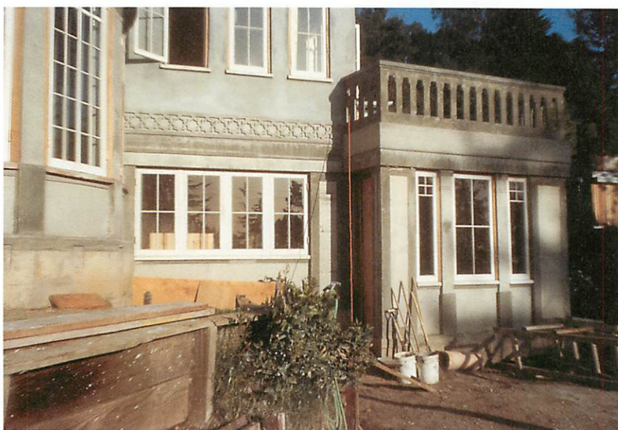
The combination of windows in the finished house, as some of them looked from the outside. The frieze and balustrade completed
