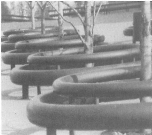
Development: Fancy railing with no purpose
