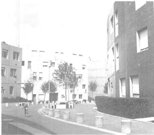
Development: Heavy-handed and authoritarian bollards and paving in developer-built place: they tell you what to do, and give no options.
