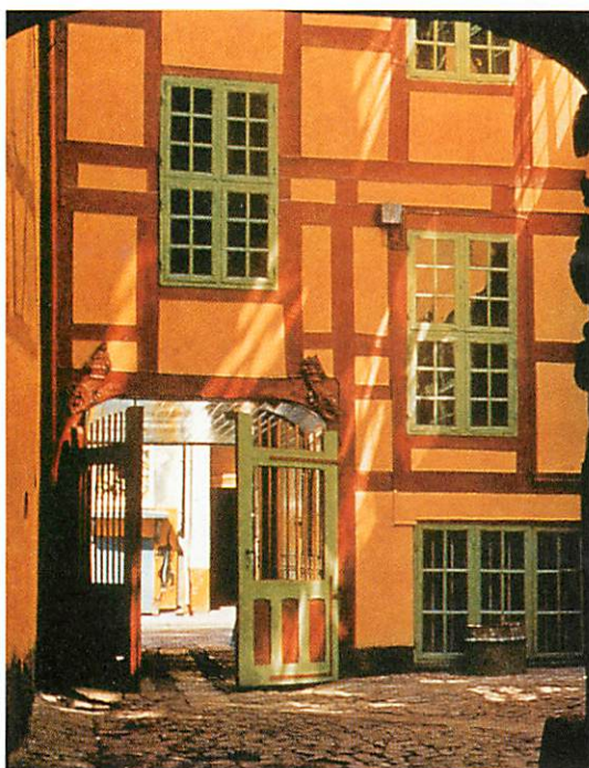
Courtyard house, Copenhagen. Here uneven, syncopated, local symmetries form a perfectly harmonious whole.
