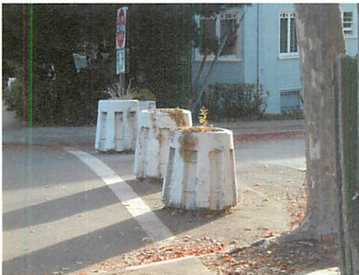
One of the traffic barriers as installed by the Berkeley Public Works department
