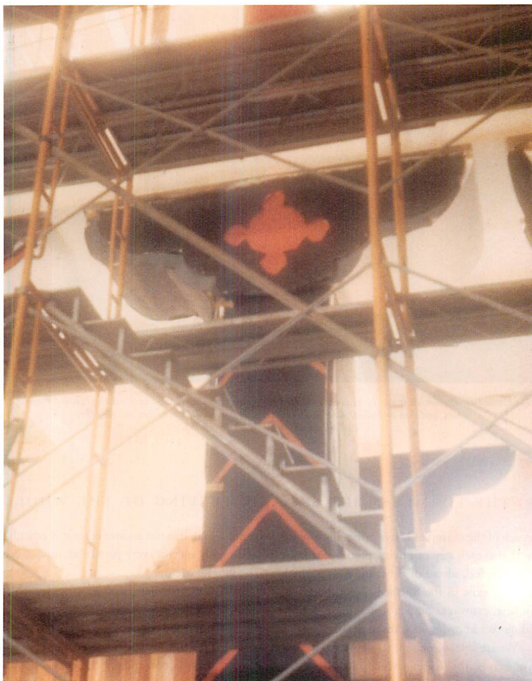
Paper-covered mockup in the Great Hall, during construction, 1985
