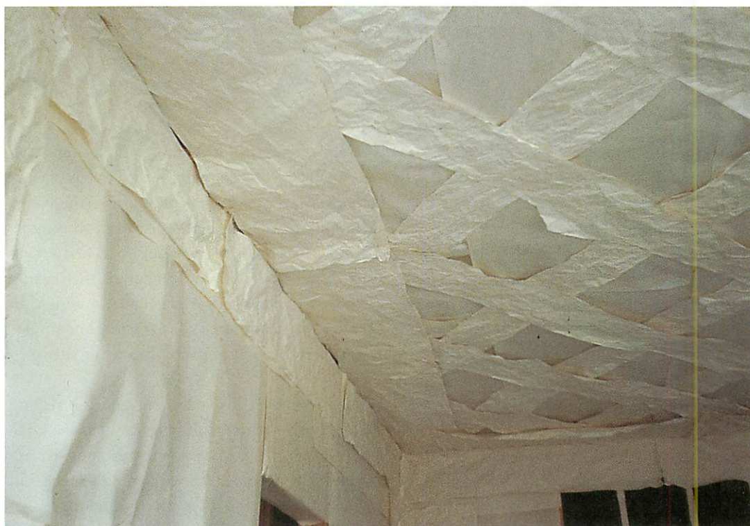
Mockup in paper to test the overall pattern of the plaster panels on the ceiling. This part concentrates on the edge, where the width of the panels had to be chosen very carefully, to get a proper harmony.
