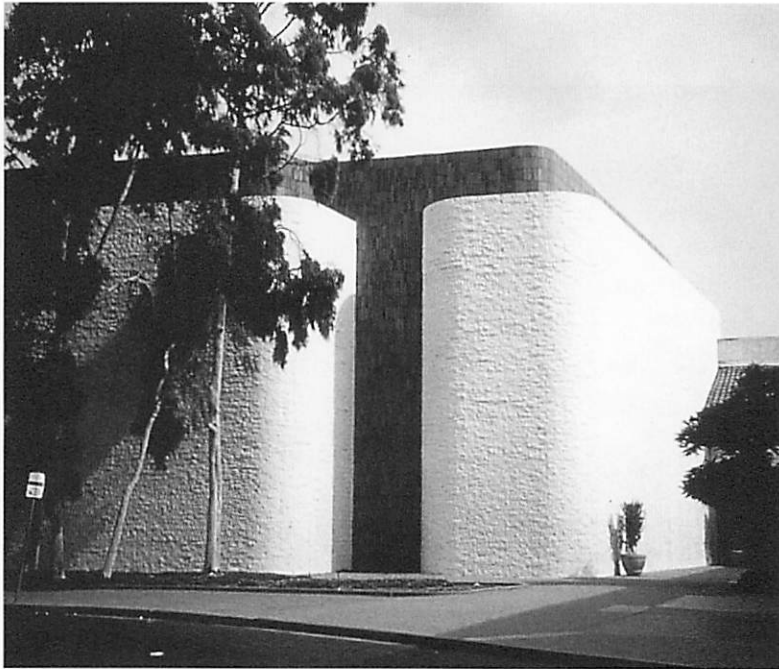
Conventional stucco bank building from southern California. Here the geometry is meaningless. Unlike the Turkish tomb on page 125, here the centers, such as they are, have not arisen naturally from the wholeness and its centers: they have merely been superimposed on the lath and plaster by the willful pencil of the architect.
