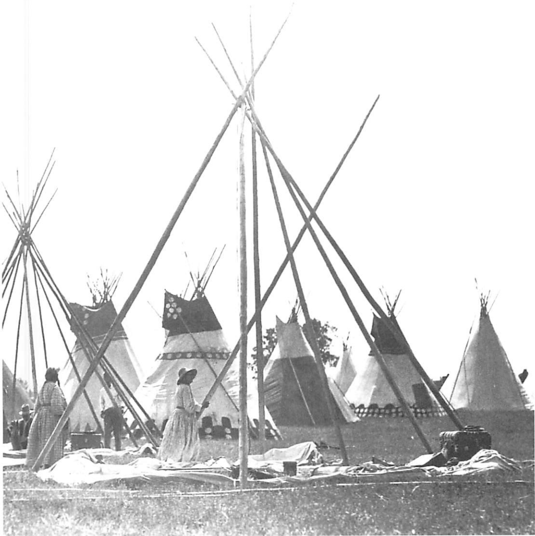
Building a tipi among the Blackfeet: The form is defined by, created by, the steps of the process.
