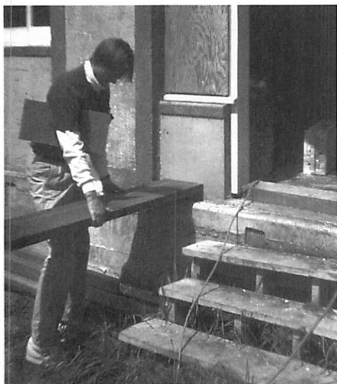
Another project, where these steps were worked into place and roughly cast, just where we wanted them, at the size we wanted them, and at the height we wanted them.
