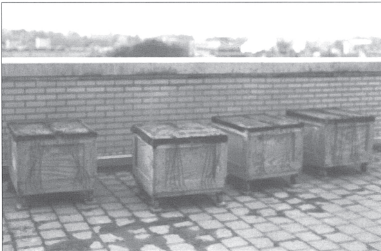
Figure 6.3 Photograph of the four soil boxes on the roof of Walker Building, Penn State University.
