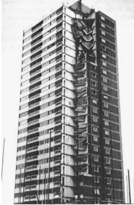
Figure 3.6 The collapse of the Ronan Point apartment complex in the United Kingdom.
