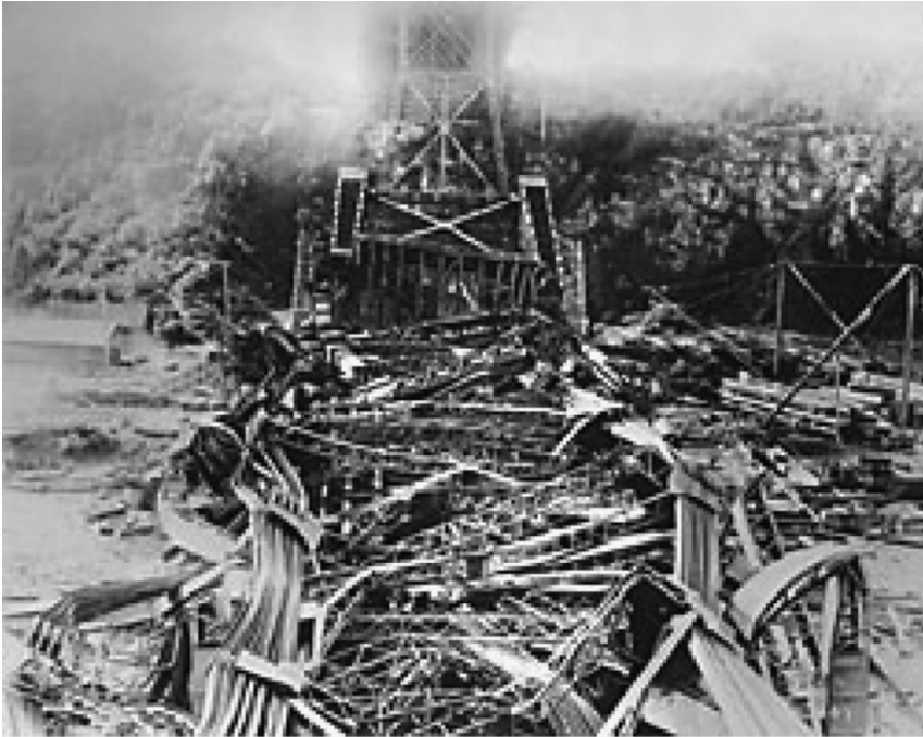
Figure 3.9 The collapsed Quebec Bridge.
