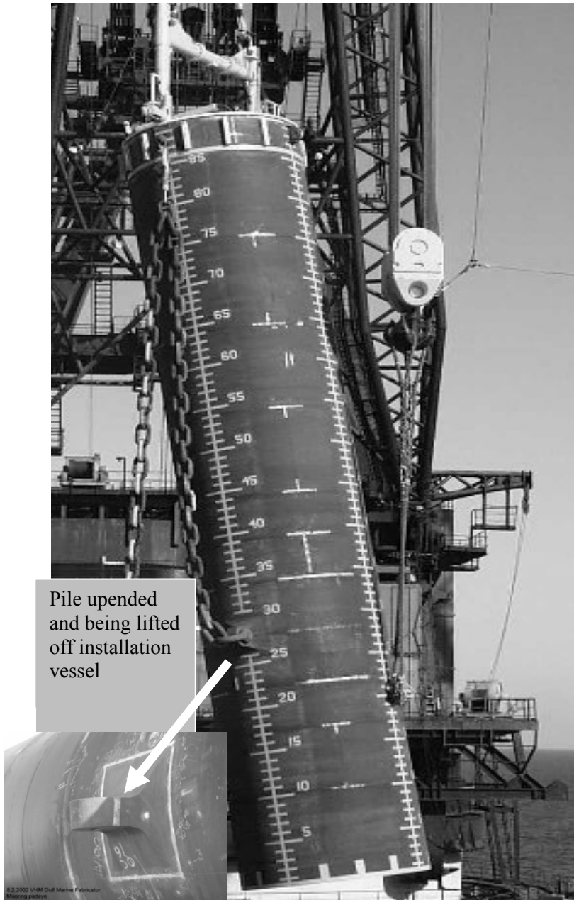
Fig. 2-13. A suction pile foundation for a spread mooring system as it is lifted
