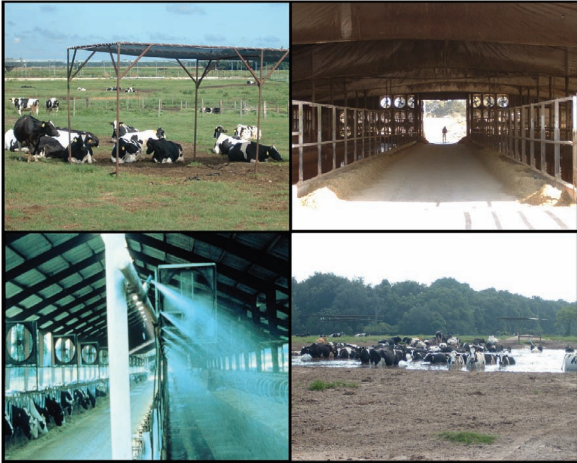
Figure 5 (see color plate 90) Some housing systems to cool dairy cattle during heat stress. The shade structure shown in the upper left panel is insufficient for adequate cooling in lactating cows. The photograph in the lower left shows a barn with sprinklers and fans installed over the feeding area. Such a system can provide significant cooling but often reproduction is still compromised during heat stress. A barn with tunnel ventilation is shown in the upper right photograph. Tunnel ventilation can be an effective system for cooling cows but is also expensive to construct. The photograph in the lower right panel shows cows cooling themselves in a man-made cooling pond. Reproduced from Horizons with permission of Genex Cooperative (2006) 12(3): 12–13.
