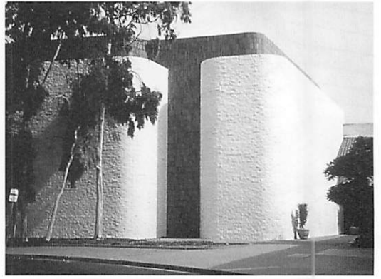
Simplified white stuccoed bank building, Southern California
