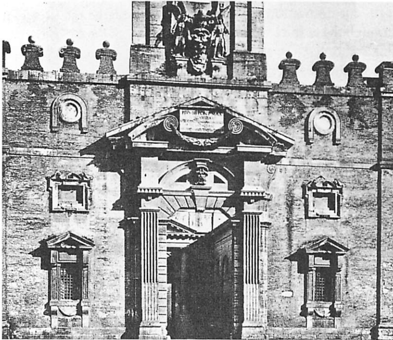
Eclectic building by Michelangelo: the ECHOES property is missing. There are far too many different morphological themes, and the composition is confusing.
