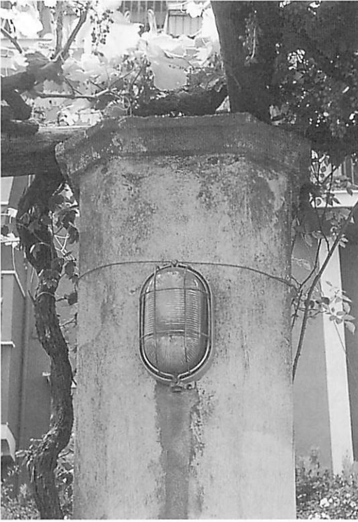
Light placed to help the top of the column
