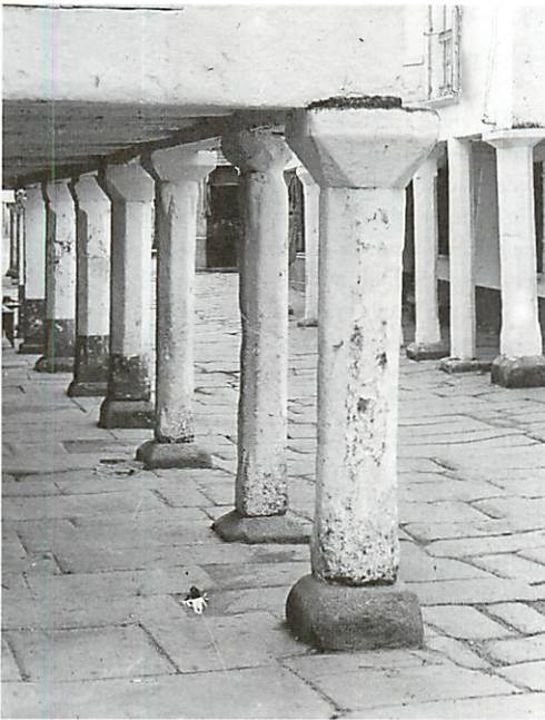
Boundary of a building made by columns and arcades. Notice how each column has its own internal boundaries at the capital and base; and how these two have their own boundaries in the line of detail which bounds them in turn.
