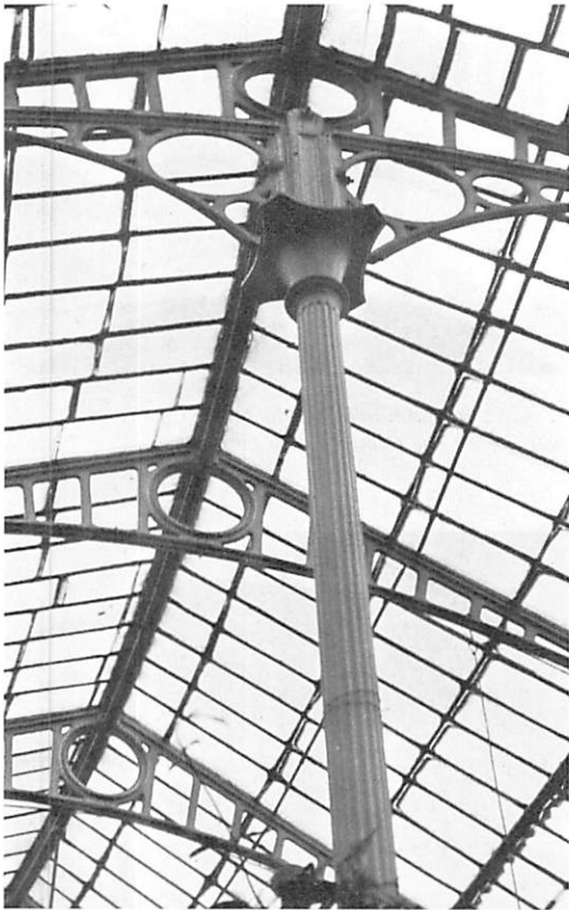
Glass and iron roof structure, London
