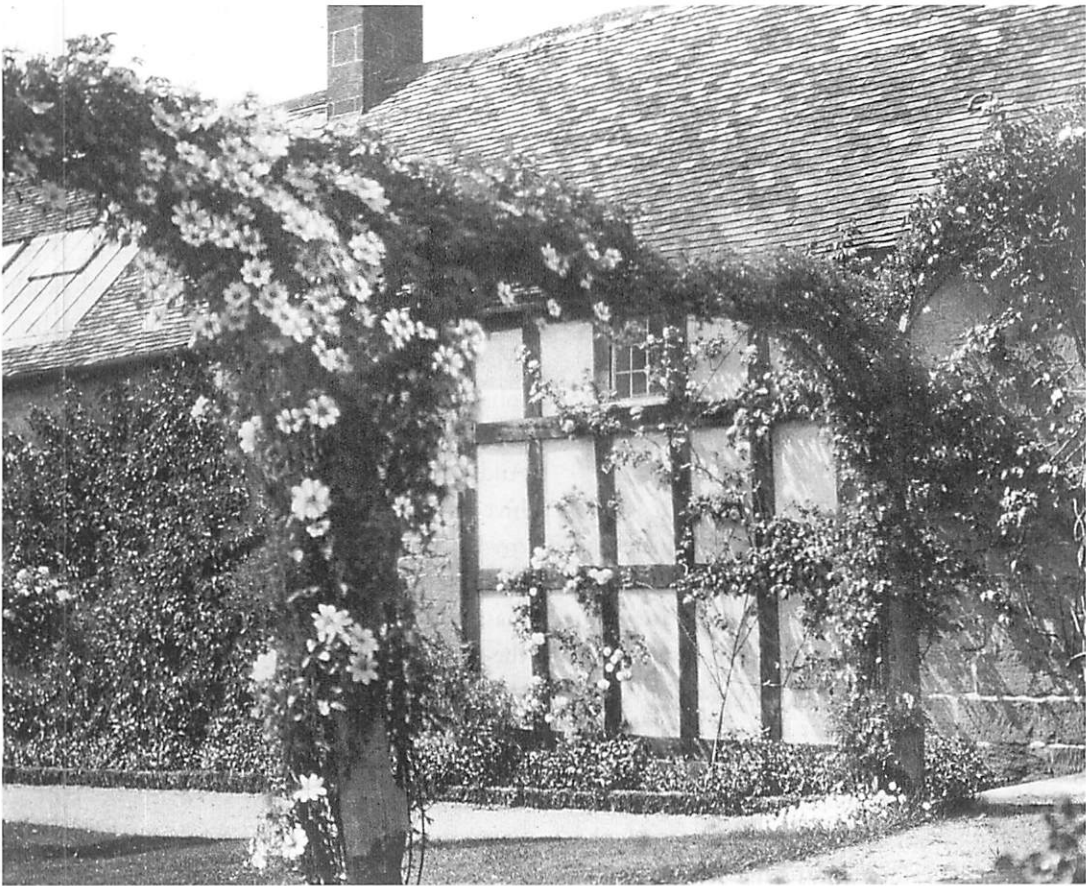
Cottage with roses: its character is given by its dominant centers, the roses, the arch of roses, the timber frame, the plaster squares.
