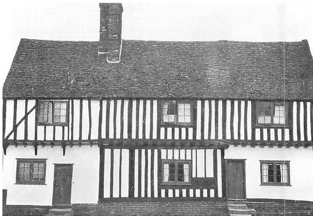
Roughness in the spacing of columns, shaping of columns, all caused by the process of construction and the detailed adaptation which has occurred.
