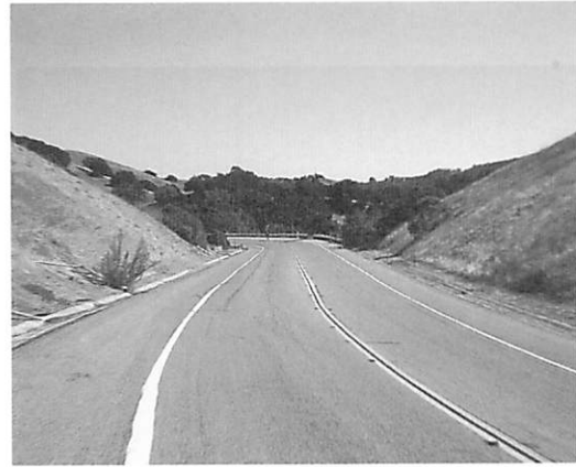
Road cut through the hills
