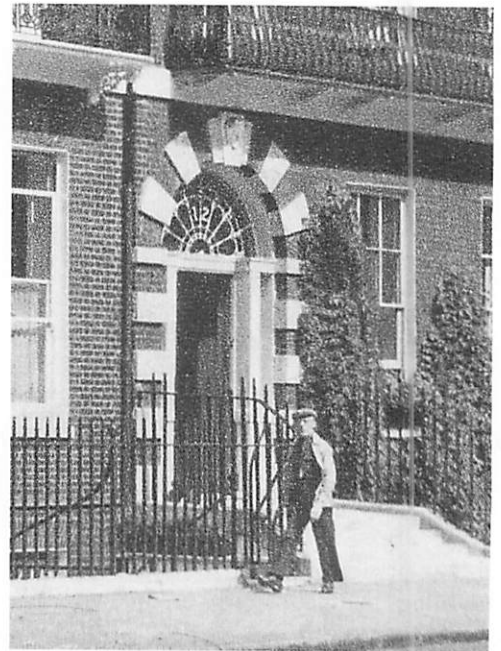
More subtle Georgian door, with a greater density of centers
