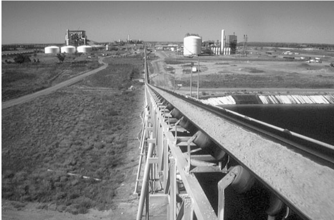
Fig. 7.4 View of parts of the fertilizer production facility at Phosphate Hill, Australia. Ammonia plant ( far right ), phosphoric acid facility ( centre ), granulation plant ( left ), and rail loadout facility ( far left ). A conveyer belt delivers phosphogypsum to the stack
