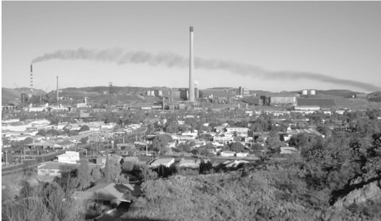
Fig. 1.11 The copper and lead smelter stacks at Mt. Isa, Australia. Until recently, the sulfurous plume was dispersed over the town and across 100,000 km 2 northwest of Mt. Isa. Over the years, the emissions resulted in the acidification of local soils and killed or reduced vegetation in the vicinity of the smelters. The recent installation of a sulfuric acid plant has reduced sulfur emissions
