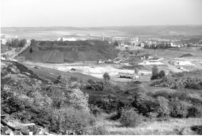
Fig. 1.9 Abandoned slag and waste heaps of copper ores, Eisleben, Germany. Mining in the area occurred for over 800 years, resulting in over 2000 individual waste heaps, 1000 km of underground workings and 56 million cubic meters of mine voids. Under the East German communist regime, the extraction of metals from very low grade, uneconomic copper ores was pursued, and large volumes of fly ashes, tailings, and smelting slags were generated. The unconstrained release of wastes into the local environment, especially of atmospheric emissions from smelting works, has caused widespread contamination of streams and lakes with metals and metalloids
