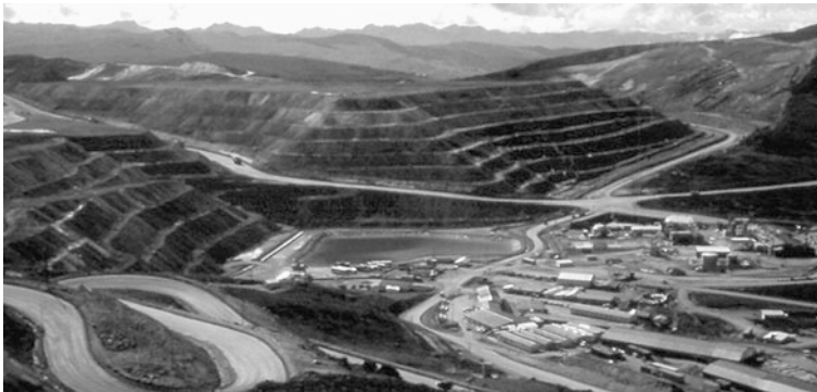
Fig. 5.5 Large heap leach piles at the Yanacocha gold mine, Peru. The siliceous gold ore is so porous that it can be heap leached without crushing. (Photo courtesy of P. Williams)
