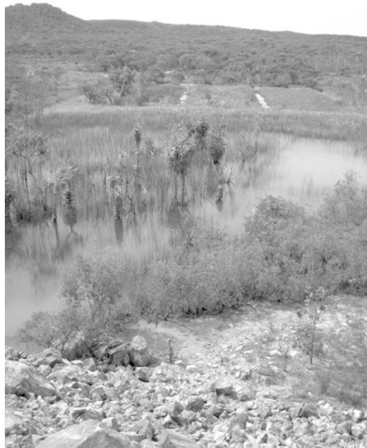
Fig. 3.28 Wetland at the Horn Island gold mine, Australia. The wetland has failed because an adjacent damwall was constructed using acid generating waste rocks (foreground), which resulted in significant AMD and caused plant death
