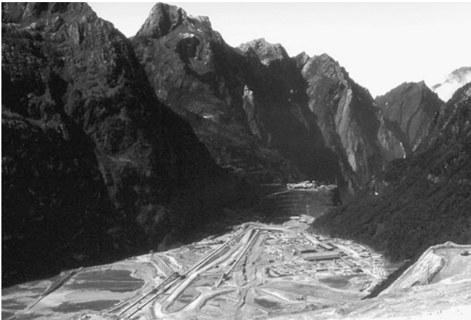
Fig. 1.10 The Ertsberg open pit, Irian Jaya, Indonesia. The Grasberg-Ertsberg mine – located at about 4000 m among the jagged alpine peaks of the Jayawijaya mountain range – is one of the world's largest mining operations. Approximately 0.24 Mt of copper ore are mined every day, and 0.2 Mt of tailings are dumped into the Ajkwa River system every day, causing increased sedimentation on the coastal floodplains
