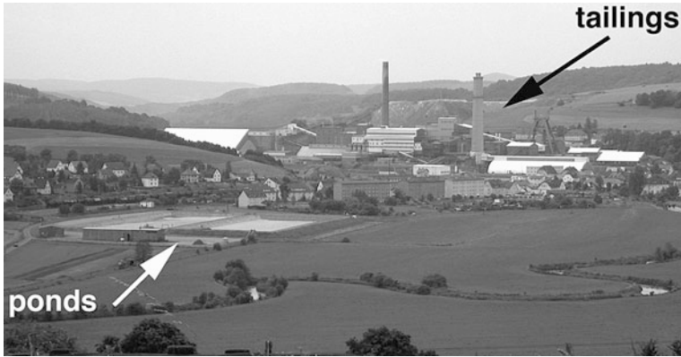
Fig. 7.1 Potash mining operations at Unterbreizbach, Germany. Dry salt tailings have been stacked into piles, and retention ponds allow the controlled release of brines into the local river
