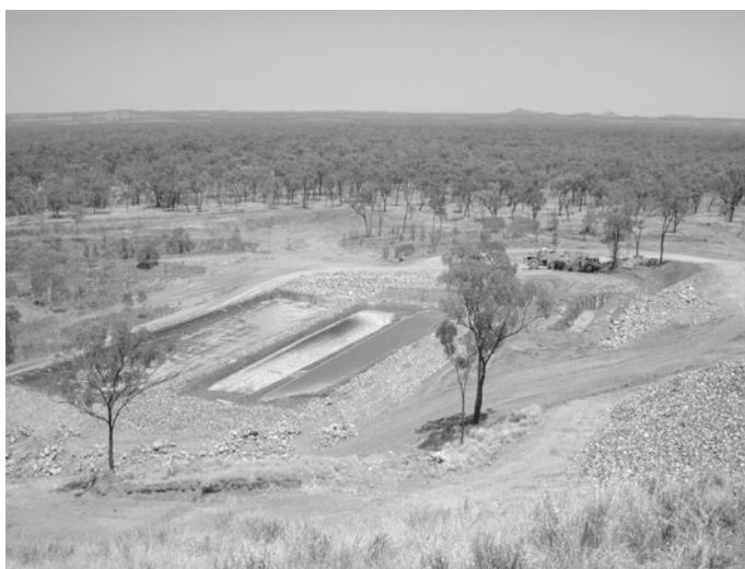
Fig. 5.8 Collection of cyanide-bearing seepage waters in shallow ponds at the base of the tailings dam, Red Dome gold mine, Australia. UV radiation causes the destruction of dissolved Cu cyanide complexes, precipitation of cyanate salts and attenuation of total cyanide from 300 \text{ mg l}^{-1} to <1 \text{ mg l}^{-1} in the successive ponds
