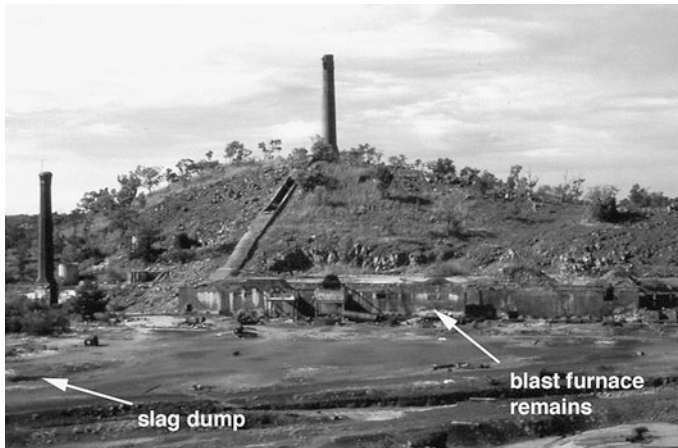
Fig. 1.5 Derelict copper-lead-gold-silver smelting works at Chillagoe, Australia. Smelting operations were conducted from 1901 to 1943 and produced 1 Mt of slag. The slag contains wt.% levels of zinc that is principally hosted by glass, olivine and hedenbergite
