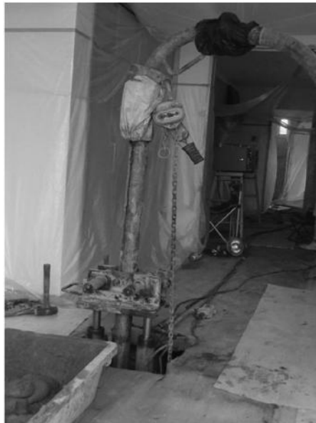
Figure 18. Compaction grouting method applied through floor of an existing house.
