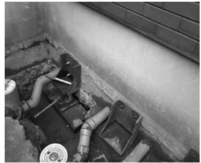
Figure 12. Lifting house superstructure with jacks.
