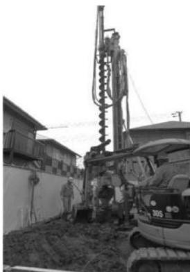
Figure 9. Compact gravel compaction with drain method applied to a house reconstruction.
