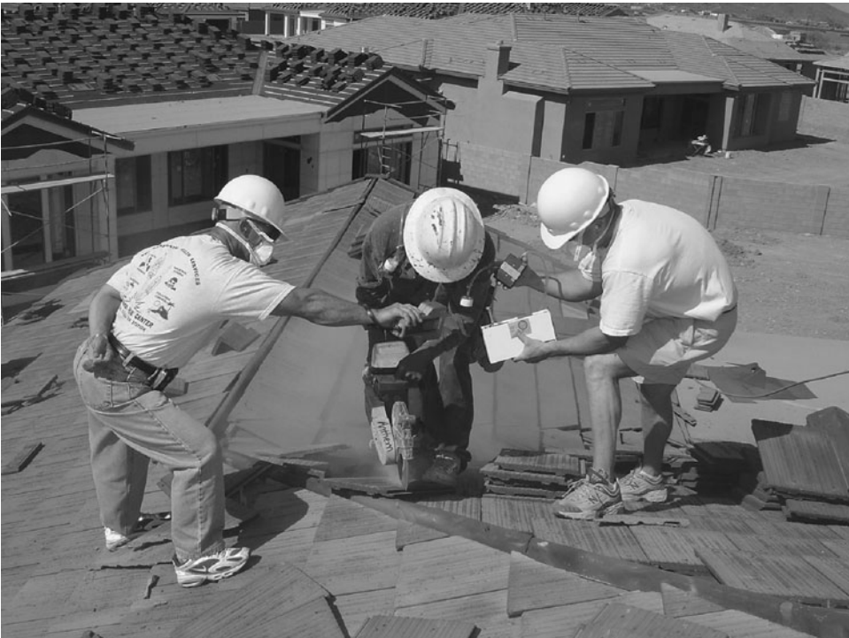
Figure 34-2. Industrial hygienists collect follow-up samples for a silica exposure among roofers. (Courtesy of the National Institute for Occupational Safety and Health.)
