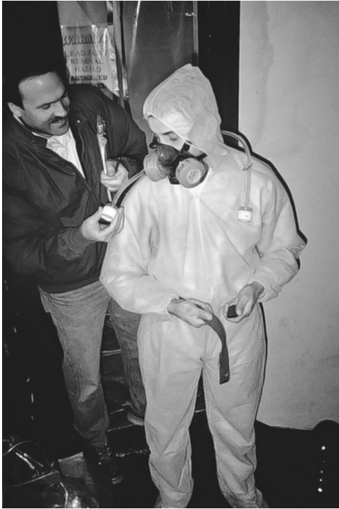
Figure 2-8. A National Institute for Occupational Safety and Health (NIOSH) industrial hygienist prepares to sample a worker’s lead exposure during a residential lead-based paint abatement project. (Photograph by Aaron Sussell.)
