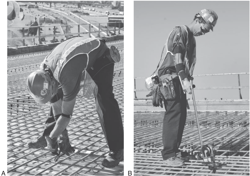
Figure 36-4. (A) Construction workers are at increased risk of upper-extremity and back strain. (B) An ergonomically designed device decreases the upper-extremity and back strain on construction workers who are tying rebar. (Photographs by Earl Dotter.)
