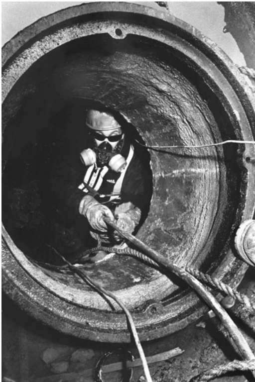
Figure 2-1. Many jobs require work in confined spaces, which requires specialized training and procedures, which are specified in the OSHA standard on Permit-required Confined Spaces (1910.146) (Photograph by Earl Dotter.)
