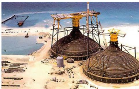
(a) – Construction on shallow dewatered basin on shore
