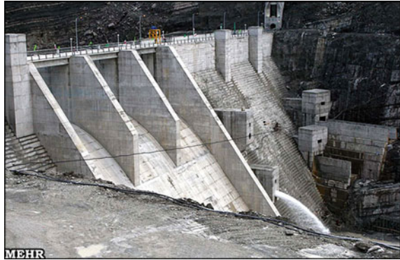
Fig. 1.28 RCC Jagin Dam in Iran
