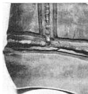
Figure 1.36 Example of 'weld decay' in an austenitic steel. (Courtesy of ICI)
