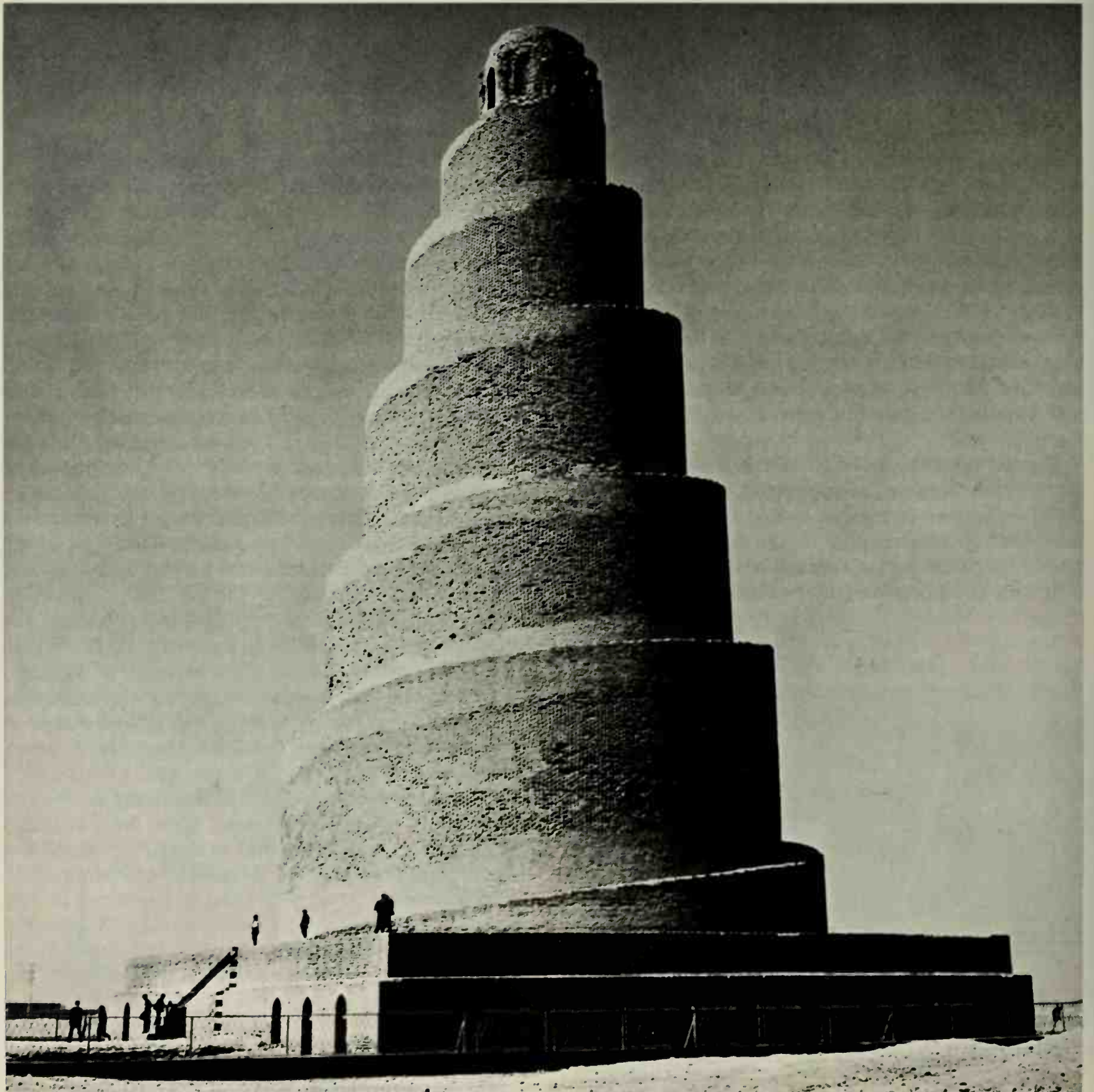
355. Spiral minaret, Great Mosque of al-Mutawakkil. Fired brick, height 176'
