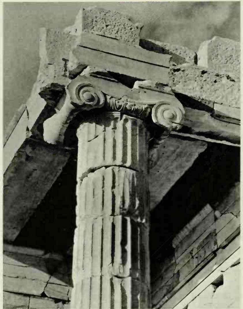
153. Ionic capital on column in central passage of Propylaea. The Acropolis, Athens
