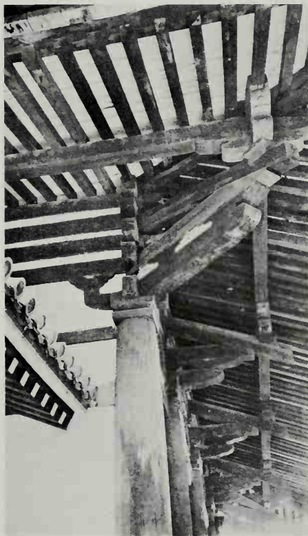
262. Hōryūji, Japan, middle gate, corner detail
