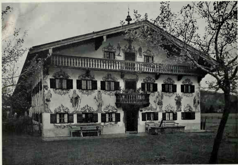
(A) Hagenberg, Jodlbauchhof, 1786, with paintings on façade
