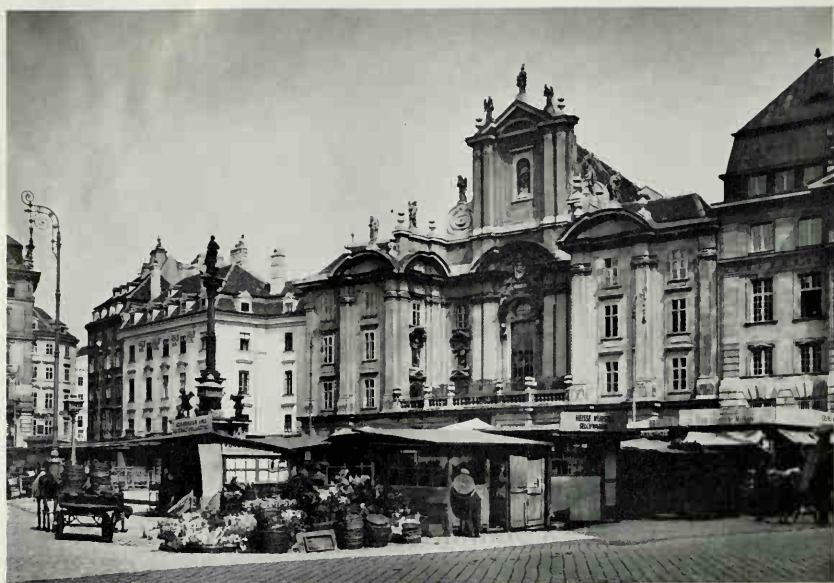
(A) Carlo Antonio Carlone: Vienna, church of the Nine Angelic Choirs, 1662. Façade
