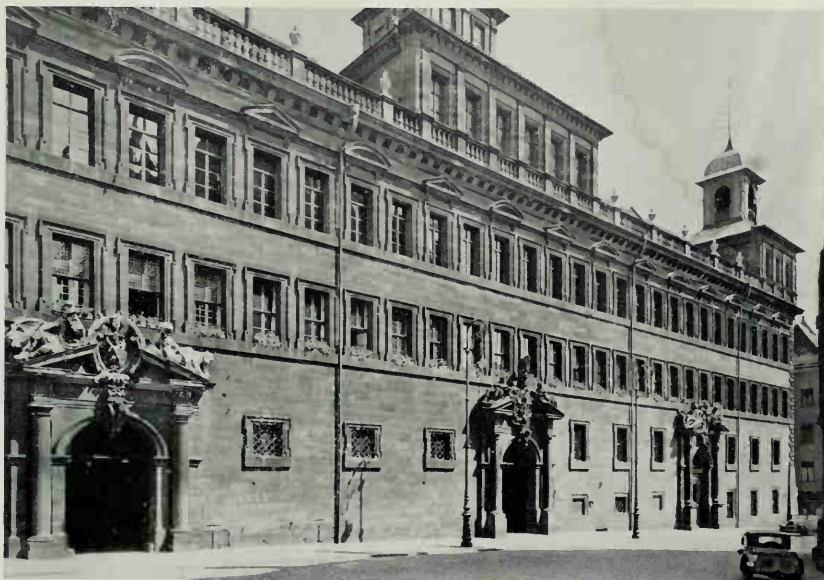
(A) Jakob Wolff the Younger: Nuremberg, additions to the town hall, 1616–22. Exterior (partly restored, destroyed in the war and since rebuilt)
