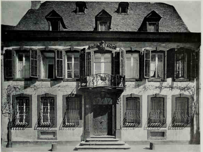
(B) Trier, No. 39 Krahenstrasse, mid eighteenth century. Façade
