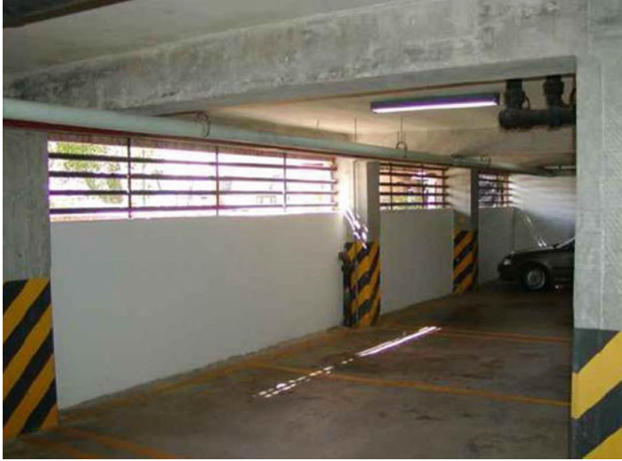
Picture 5.7 Part height wall in few bays – short columns formed
