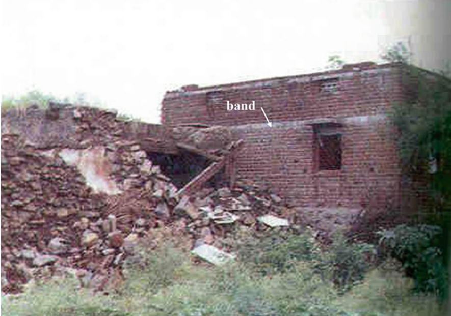
Picture 9.4 Benefit of using confining bands
