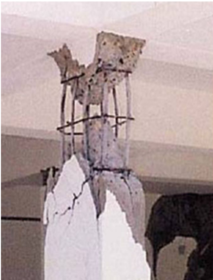
Picture 6.6 Column failures
