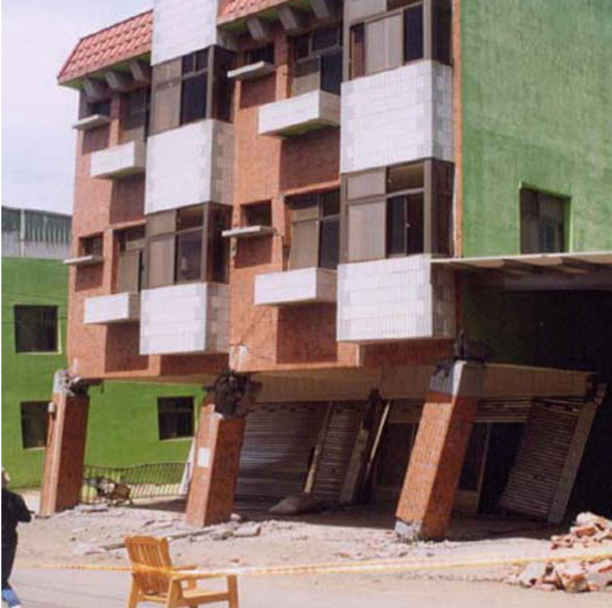
Picture 6.4 Storey sway mechanism
