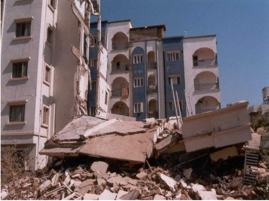
Picture 6.2 Progressive-type failure
