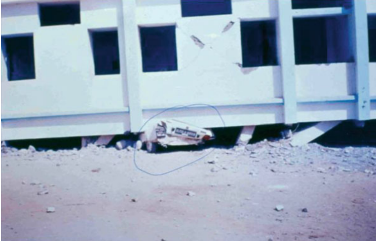
Picture 5.5 Collapse of a soft storey
