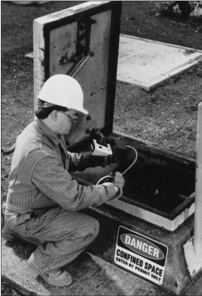
Figure 17-8. A worker cautiously monitors a confined space in order to evaluate its atmosphere. (Courtesy Draeger Safety, Inc.)
