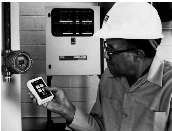
Figure 18–3. This multipoint ambient air monitor is capable of continually measuring up to five gases in as many as 24 remote locations. (Courtesy MSA.)
