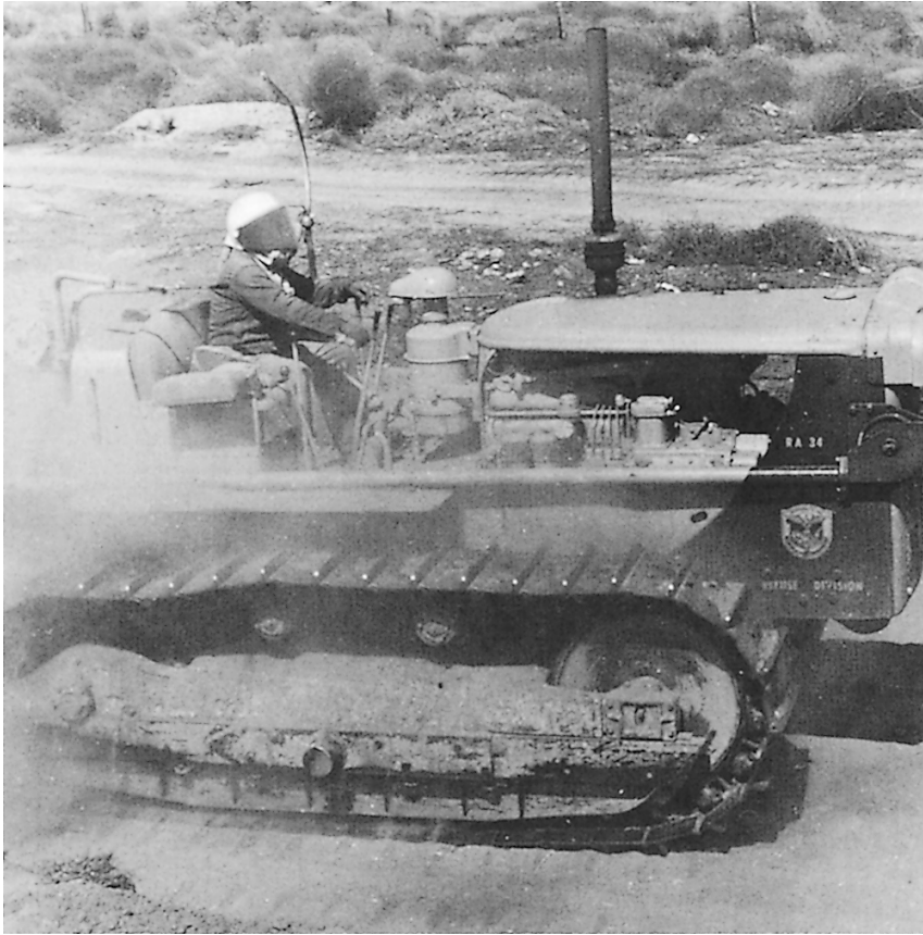
Figure 18–13. This operator is provided with clean, respirable air.
