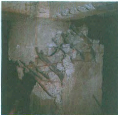
Photo 2-20: Thin widely-spaced plain bars were used as lateral reinforcement in columns failing in shear. (Left): in Baguio, the 1990 Luzon Earthquake, Philippines, (Right): in 1986 Kalamata earthquake, Greece.
