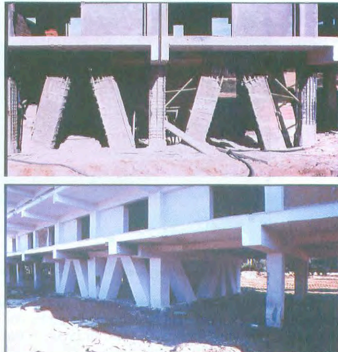
Fig. 5-38: Foundation of new wall through diagonal concrete braces: (a) transfer of wall forces to ground; (b) shotcreting of braces and of columns jackets; (c) retrofit completed.
