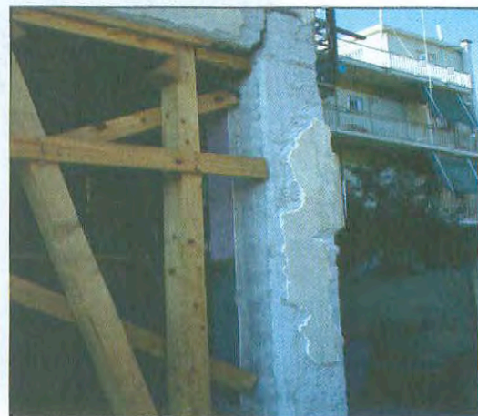
Photo 2-26: (Left) No lateral reinforcement was placed in a beam-column joint; the column longitudinal reinforcement failed in splitting of plain concrete in the anchorage region due to lack of confinement. (Right) Separation of beam from corner joint in the 1986 Kalamata earthquake, Greece, due to short straight anchorage of beam bars in the joint.
