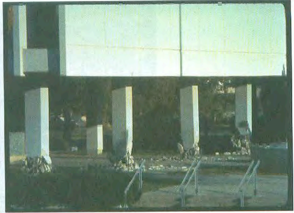
Photo 2-1: Imperial County Services Building damaged in the 1979 Imperial Valley earthquake. Source: National Information Service for Earthquake Engineering (NISEE), Univ. of California, Berkeley.
