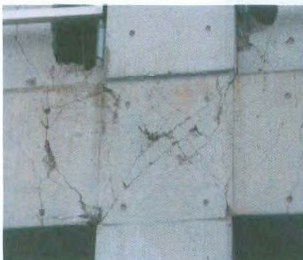
Photo 2-27: (Left) Beam-column joints of weak-beam strong-column building were heavily cracked in shear during the 1995 Hyogo-ken Nanbu, Japan earthquake. (Centre) Joint failures in older concrete frame in 1994 Northridge earthquake. Source: NISEE (Right) Diagonal failure of unreinforced corner column in 7-storey building in the 1986 Kalamata earthquake, Greece.
