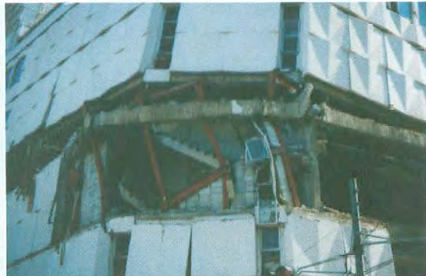
Photo 2-14: (Left) Damage of an entrance door and non-structural concrete partition walls due to large deformation in the 1995 Hyogo-ken Nanbu (Kobe) Earthquake, Japan. (Right) Fallen heavy precast concrete curtain walls in a building, Kobe City, in the 1995 Hyogo-ken Nanbu (Kobe) Earthquake
