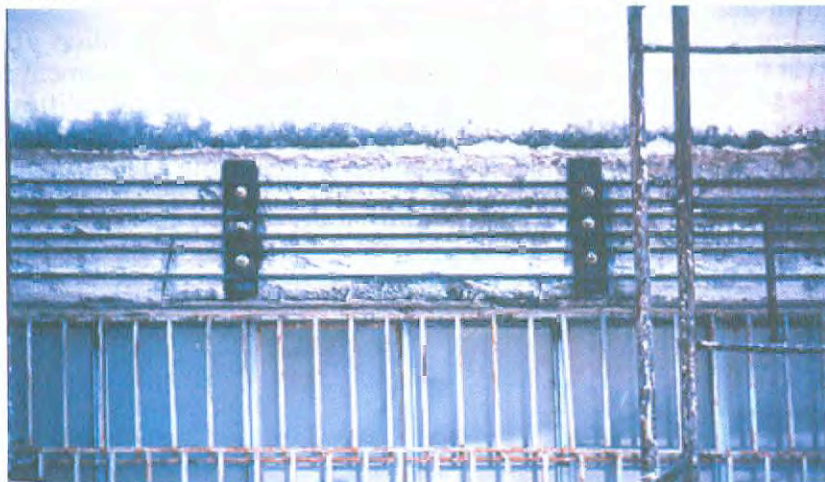
Fig. 5-36: Collector element for concrete walls of Fig. 5-35, fastened to side of perimeter beams.
