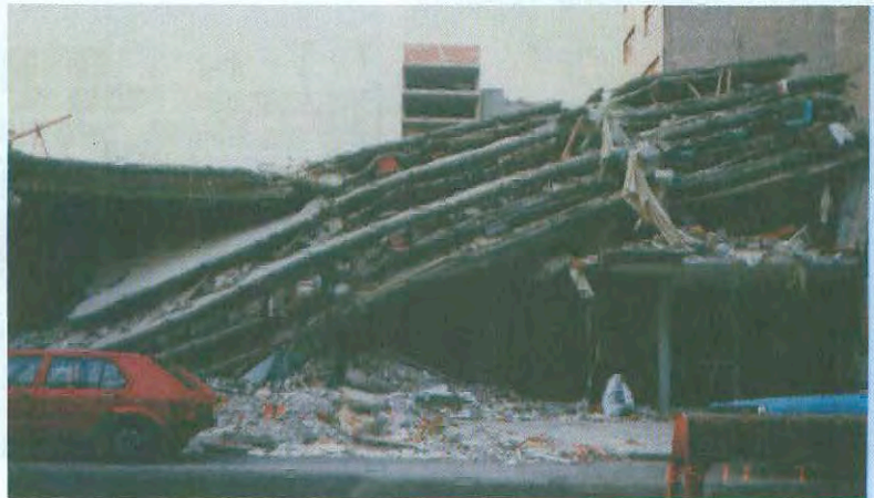
Photo 2-13: Failure of a school building in Mexico City during the 1985 Mexico earthquake. Many buildings failed in the pancake failure mode.
