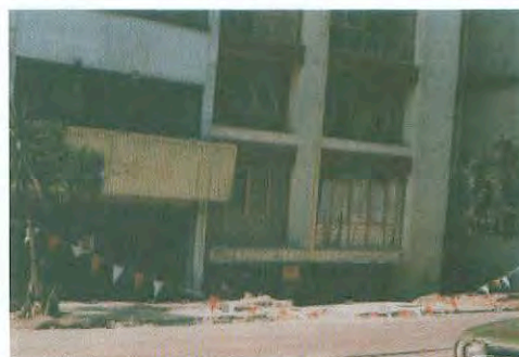
Photo 2-15: (Left) Overturned apartment buildings, Niigata City, due to liquefaction of sandy soil in 1964 Niigata Earthquake, Japan. (Right) Settlement of buildings due to liquefaction of soil in Mexico City during the 1985 Mexico Earthquake, Mexico.
