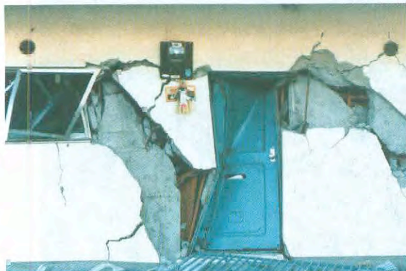
Photo 2-14: (Left) Damage of an entrance door and non-structural concrete partition walls due to large deformation in the 1995 Hyogo-ken Nanbu (Kobe) Earthquake, Japan. (Right) Fallen heavy precast concrete curtain walls in a building, Kobe City, in the 1995 Hyogo-ken Nanbu (Kobe) Earthquake
