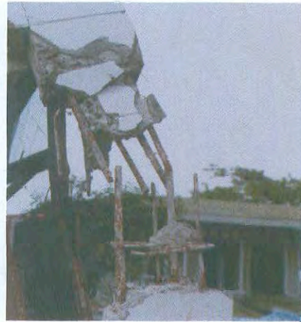
Photo 2-25: (Left) Gas pressure welding splice was fractured during the 1995 Hyogo-ken Nanbu Earthquake, Japan. (Right) Failure at lap splice in a building in Baguio during the 1990 Luzon Earthquake.
