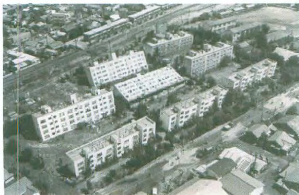
Photo 2-15: (Left) Overturned apartment buildings, Niigata City, due to liquefaction of sandy soil in 1964 Niigata Earthquake, Japan. (Right) Settlement of buildings due to liquefaction of soil in Mexico City during the 1985 Mexico Earthquake, Mexico.
