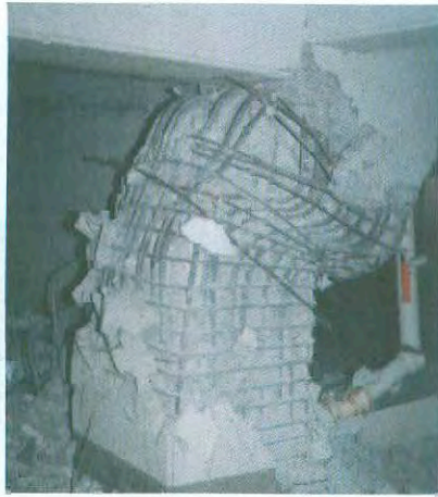
Photo. 2-18: Flexural compression failure of columns in 1995 Kobe earthquake. Column had peripheral ties at 100mm centres in Motoyama Royal Condominium Building.
