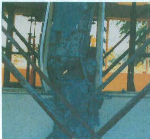
Photo 2-21: Column shear failures: (Left) in school building in Lazaro Cardenas, Mexico, during 1985 Mexico Earthquake. Spacing of the large-diameter ties was almost as wide as width of the column. Spalling of concrete was observed along longitudinal bars. (Right) in a building in 1986 Kalamata Earthquake, Greece; stirrups of plain bars were open and had no hooks or bents at the ends.
