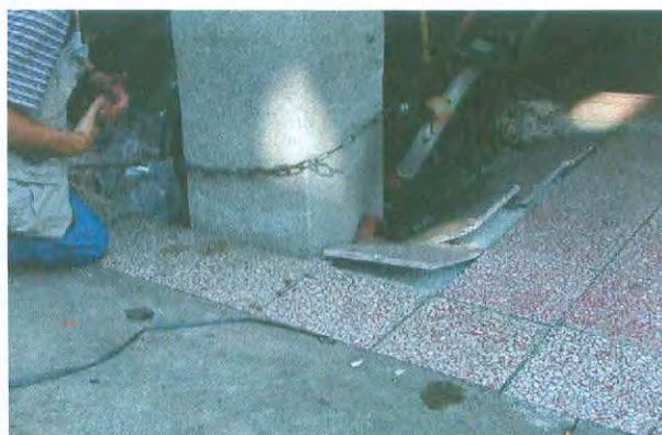
Photo 2-17: Compaction under low-rise building in 1999 Chi-Chi earthquake. Lack of evidence of liquefaction and presence of large cobbles in subgrade suggests damage due to settlement. Source: NISEE
