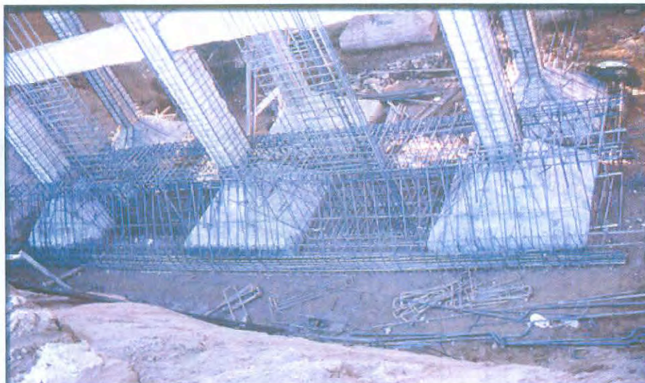
Fig. 5-36: Collector element for concrete walls of Fig. 5-35, fastened to side of perimeter beams.
