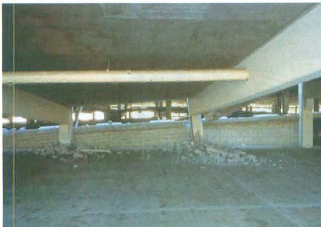
Photo 2-9: Consequence of column failures; (Left) Failure of interior "gravity" columns apparently led to (Right) progressive collapse of perimeter lateral force resisting system. 1994 Northridge earthquake. Source: NISEE
