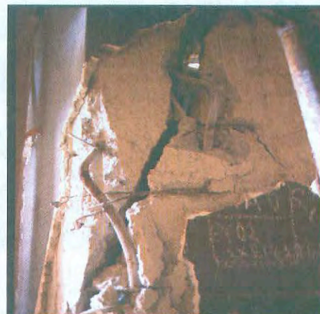
Photo 2-20: Thin widely-spaced plain bars were used as lateral reinforcement in columns failing in shear. (Left): in Baguio, the 1990 Luzon Earthquake, Philippines, (Right): in 1986 Kalamata earthquake, Greece.
