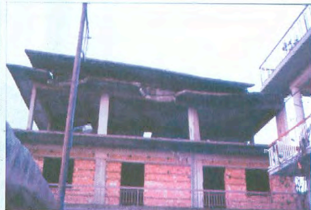
Photo 2-5: (Left) Collapse at third storey in 4-storey building in the 1999 Kocaeli earthquake in Turkey. (Right) Penthouse collapse in 5-storey building in the 1986 Kalamata earthquake in Greece.
