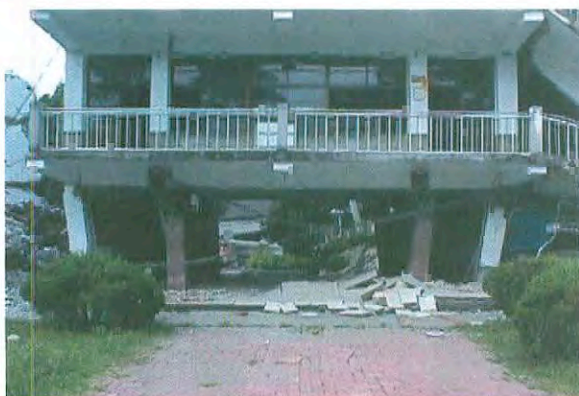
Photo 2-16: Fault rupture at building during 1999 Chi-Chi, Taiwan earthquake resulting in foundation compression, forcing columns inward. Source: NISEE
