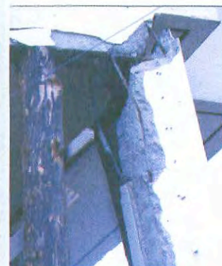
Photo 2-27: (Left) Beam-column joints of weak-beam strong-column building were heavily cracked in shear during the 1995 Hyogo-ken Nanbu, Japan earthquake. (Centre) Joint failures in older concrete frame in 1994 Northridge earthquake. Source: NISEE (Right) Diagonal failure of unreinforced corner column in 7-storey building in the 1986 Kalamata earthquake, Greece.
