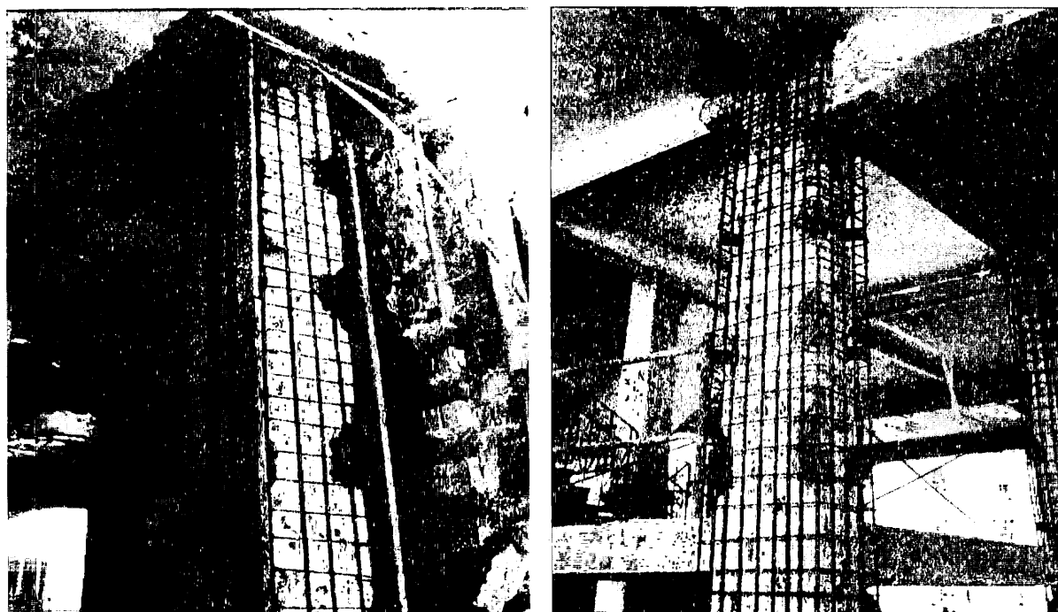
Fig. 5-3: Concrete jackets with U-shaped rebars or steel plates welded to old and new corner bars for shear connection
