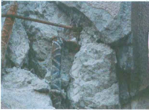
Photo 2-25: (Left) Gas pressure welding splice was fractured during the 1995 Hyogo-ken Nanbu Earthquake, Japan. (Right) Failure at lap splice in a building in Baguio during the 1990 Luzon Earthquake.
