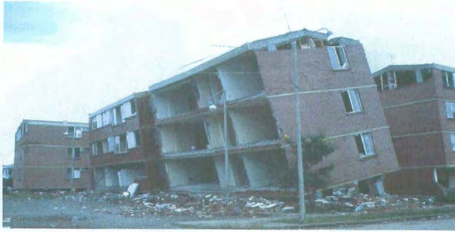
Photo 2-10: Twelve identical buildings collapsed when first storey stiff brittle masonry walls failed thus causing the reinforced concrete frame columns to fail in shear during the Popayan, Colombia, Earthquake of March 31, 1983.
