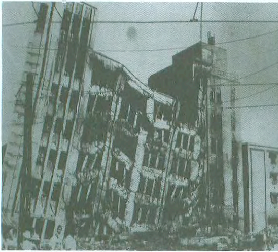
Photo 2-11: Daiwa department store building collapsed in the 1948 Fukui Earthquake. Building suffered fire before the earthquake. Soft soil condition and inadequate reinforcement details also may have contributed to the failure.
