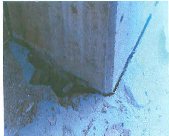
Photo 2-8: (Left) Buckled topping slab on precast diaphragm during the 1994 Northridge Earthquake. The mild tension reinforcement apparently yielded due to diaphragm flexure, then buckled as the unbonded prestressing reinforcement compressed the elongated mild reinforcement. (Right) Fractured diaphragm reinforcement at connection with structural wall. Source: W.G. Corley
