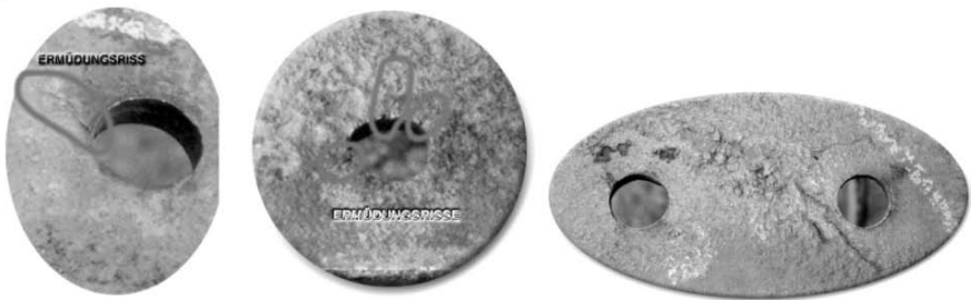
Figure 17. Cracks in elements.
