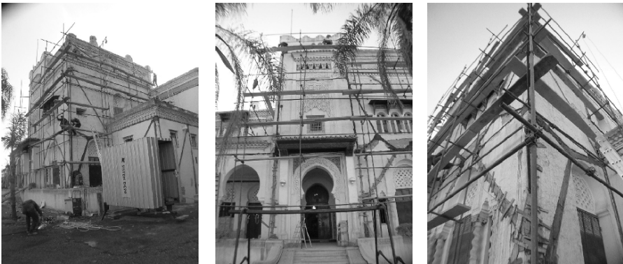
Figure 16. View of residency of Finland ambassador in Algeria under retrofitting.
