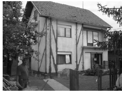
Figure 15. Experimental testing of retrofitted building.
