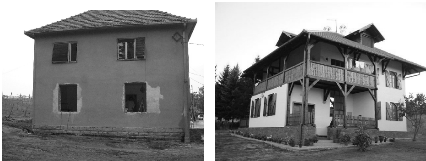
Figure 17. Experimentally reconstructed house, Lazić property (left) and strengthen object (right).
