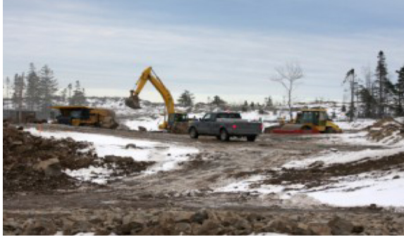
Figure 3.1 A typical construction site.
