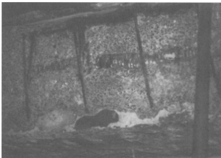
Figure 15-20. Grouted beam tendon encased by sheet metal duct.
