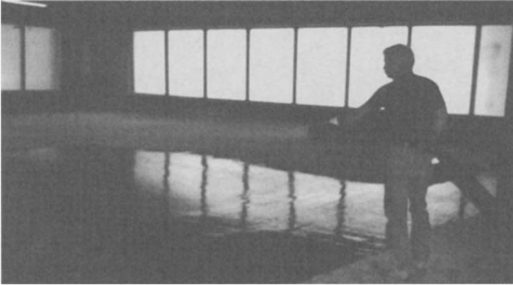
Figure 15-66. Membrane installation: Aggregates being broadcast on recently placed membrane.
