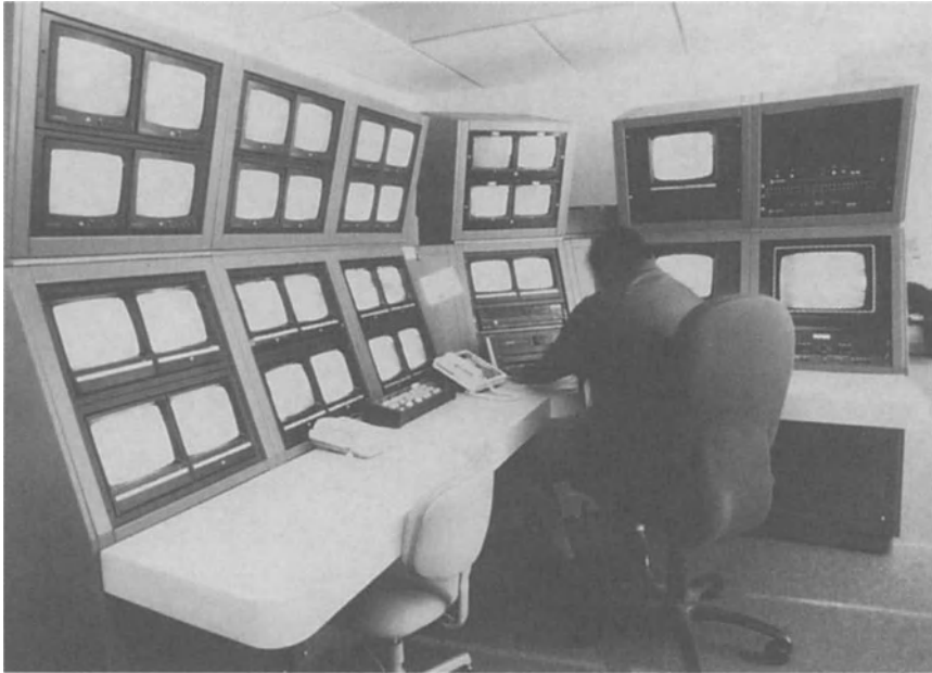
Figure 4-7. A console for monitoring CCTV coverage. Photo courtesy Duke University Medical Center.
