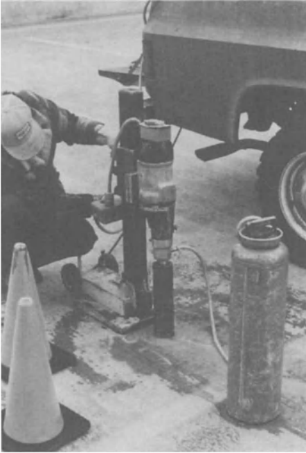
Figure 15-49. Coring for concrete samples.
