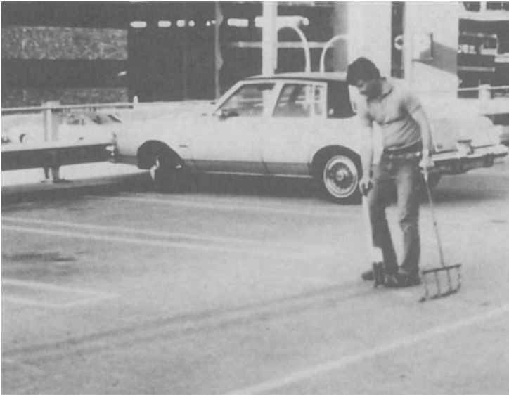
Figure 15-43. Chain drag delamination survey.
