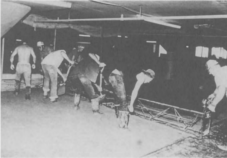
Figure 15-68. Concrete overlay placement with vibratory screed.
