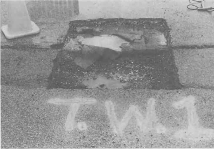
Figure 15-54. Test well to observe condition of waterproofing system and underlying concrete.
