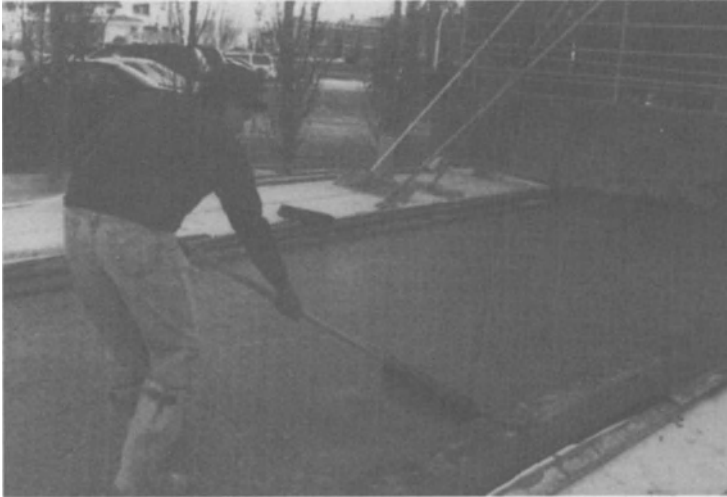
Figure 15-61. Application of bonding grout precedes concrete overlay placement.
