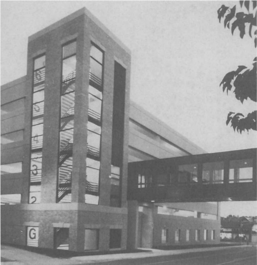
Figure 4-2. Glassback elevators and glass walls in stair towers provide visibility when these spaces must be enclosed. Photo courtesy Walker Parking Consultants.
