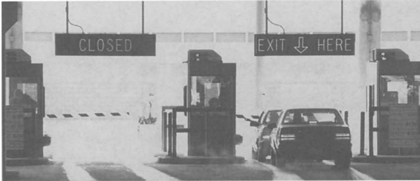
Figure 6-3. Fiber optic signs can compensate for overillumination behind the sign. Photo courtesy C. J. Hood Company.
