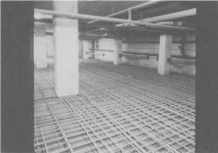
Figure 15-88. Full-depth slab replacement for long-term life expectancy.
