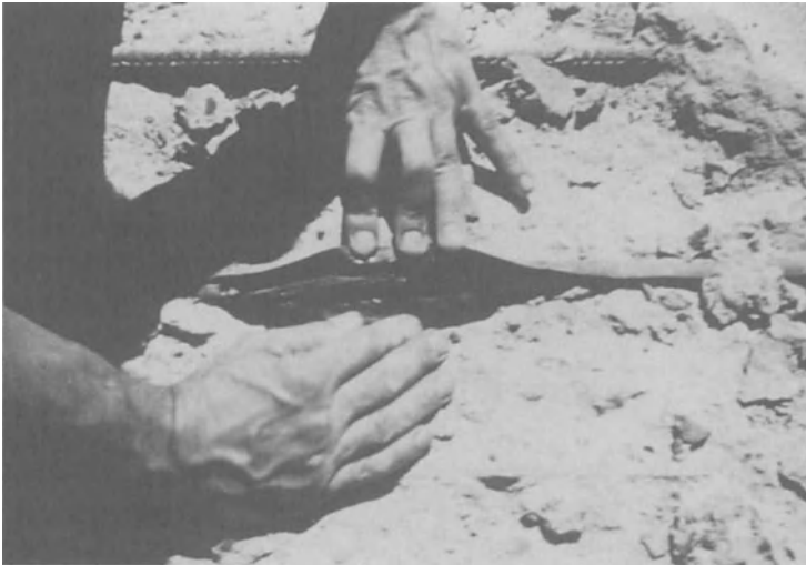
Figure 15-19. Strand with grease and push-through sheathing.
