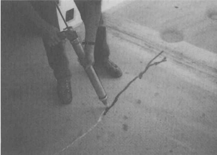
Figure 15-75. Routed and sealed random cracks.
