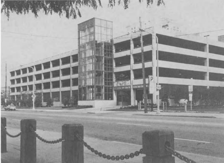
Figure 4-3. Security screening can be unobtrusive but provide control of the facility perimeter. Photo courtesy Walker Parking Consultants.
