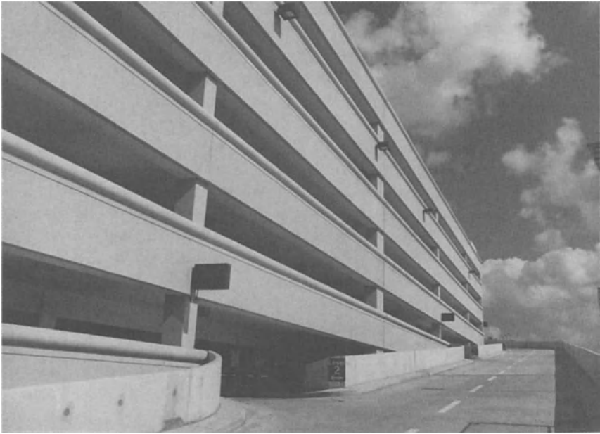
Figure 2-15. With an express ramp and flat floors, a mega-structure becomes a series of parking lots stacked vertically. Courtesy of Walker Parking Consultants.
