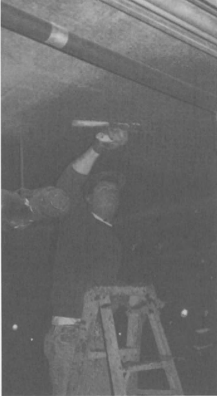
Figure 15-82. Overhead patching.
