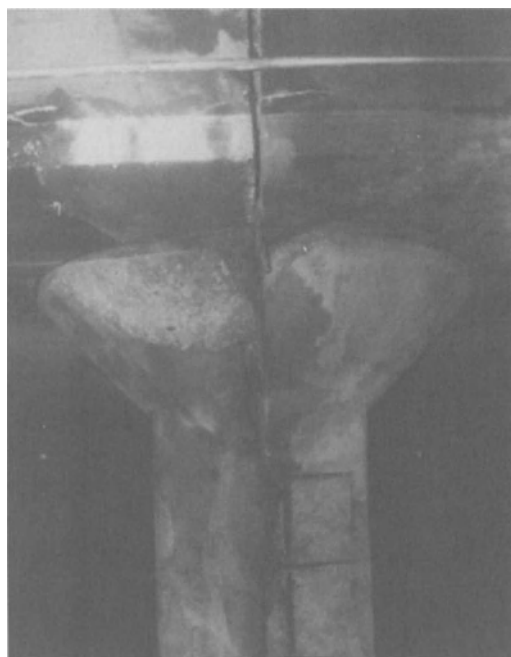
Figure 15-38. (Continued) (c) Underlying structural member deterioration due to leakage at expansion joint.
