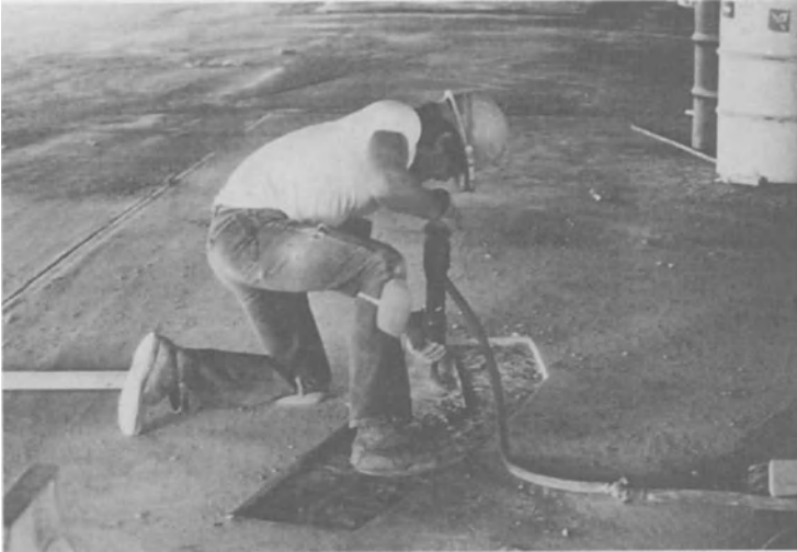
Figure 15-59. Concrete removal prior to patching floor spall.
