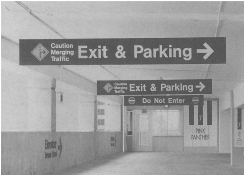
Figure 6-2. White copy on black background is very effective in parking structures. Photo courtesy Standard Parking Corporation, US Patent No. 4,874,937.
