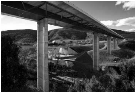
Figure 1: Partial view of the finished bridge (Photo: Paco Gómez).
