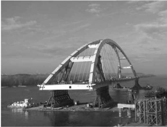
Figure 11: Erection of the arch bridge.
