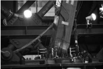
Figure 5: Local buckling of the first-story column at the end of the tests.
