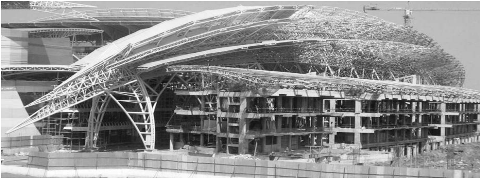
Figure 12: Central Spine under construction
