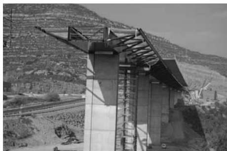
Figure 4: Stages of bridge girder construction.
