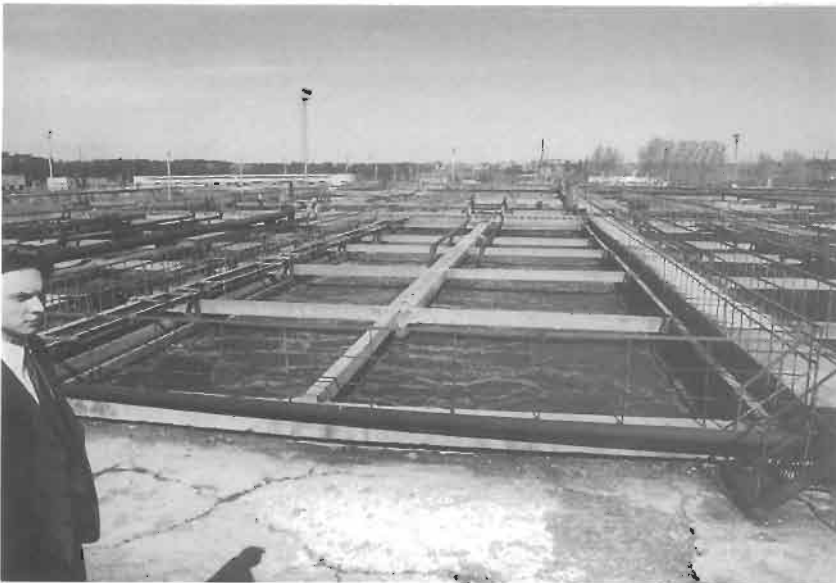
Figure 8. Rectangular settling basins in operation.
