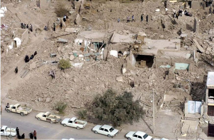
Fig. 4.7 The extent of destruction of the Bam urban fabric around the ancient citadel after the earthquake. Source HFIR (Reprinted with permission)
