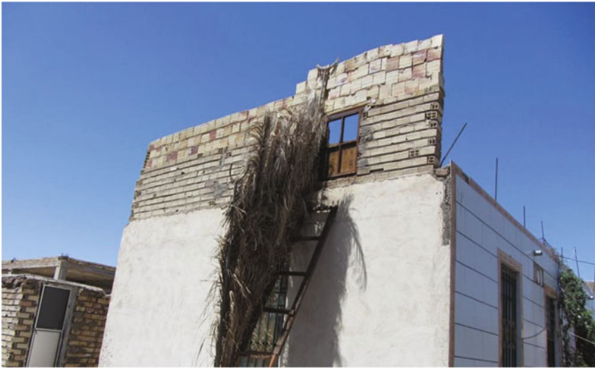
Fig. 8.5 Attaching additional elements to reconstructed houses. Photo Arefian 2013
