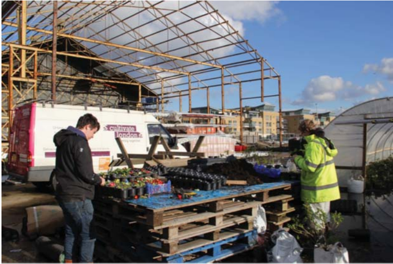
Figure 5.10 Apprentices working on site.
