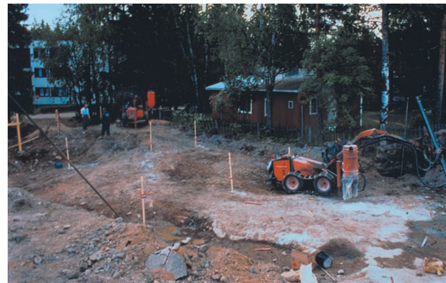
FIGURE 5.1.-2. Foundation preparation by TAMROCK Commando 100.
