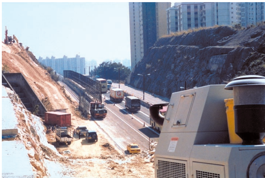
FIGURE 5.1.-1. A typical construction project- Tve Mun Highway expansion in Hong Kong.
