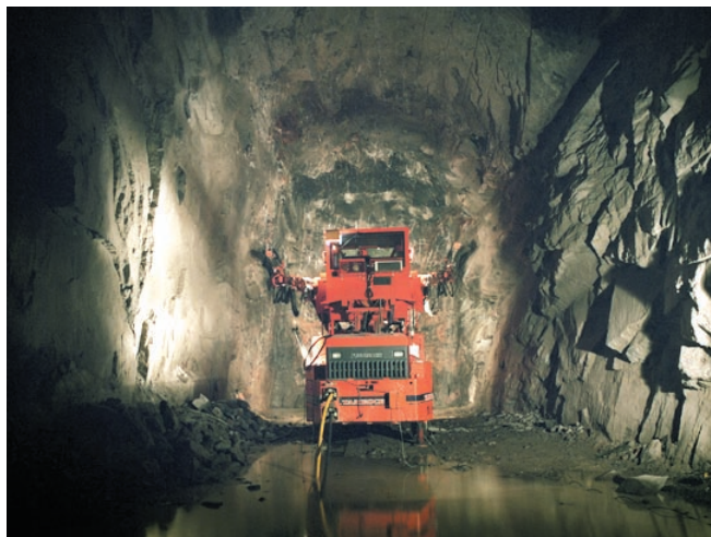
FIGURE 6.3.-1. TAMROCK Data Titan in the Norrala tunnel.
