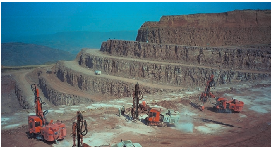
FIGURE 5.3.-3. TAMROCK bench drilling rigs at work in Xiaolangdi.
