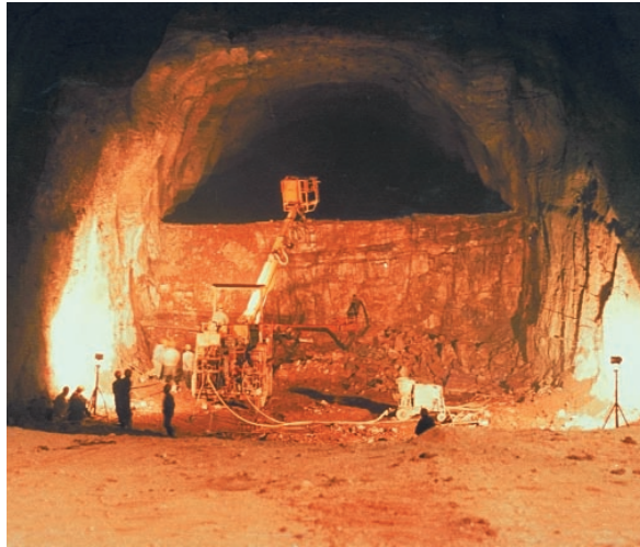
FIGURE 6.3.-3. Underground excavations in Xiaolangdi.
