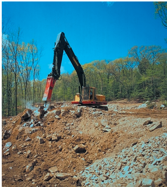
FIGURE 4.2.-44. Rammer G100 hydraulic hammer at granite quarry.
