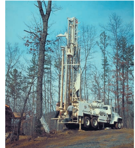
FIGURE 8.2.-5. Hydraulic top-drive air drilling rig.
